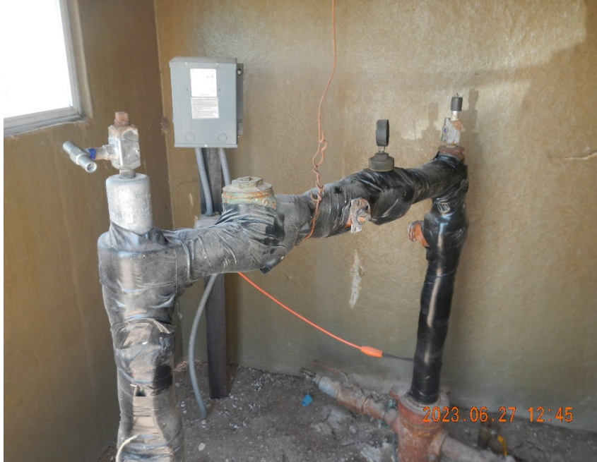
3. View of top of well.
