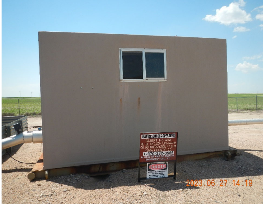
7. View of exterior at injection equipment building.
