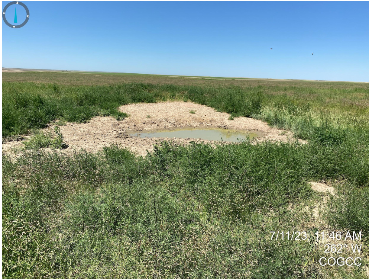
Photo 1. The former well location does not appear to have been reclaimed with the presence of gravel, undesirable vegetation (russian thistle and kochia), and the location does not appear to have been contoured or graded to reflect adjacent areas.
