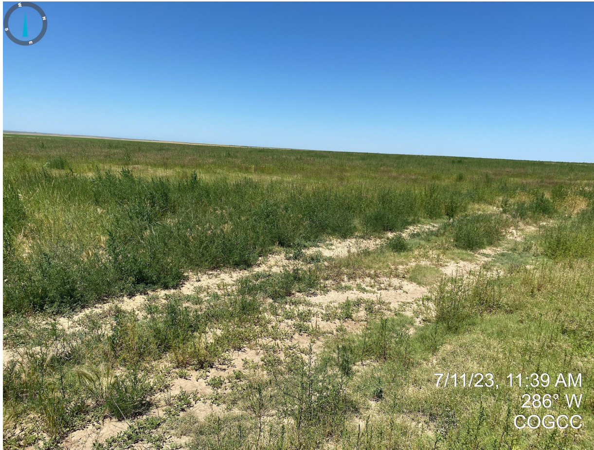
Photo 33. Taken from the reclaimed location, facing west towards the southern access road. The access road does not appear to have been reclaimed; further reclamation activities are required in order to meet Rule 1004 standards.
