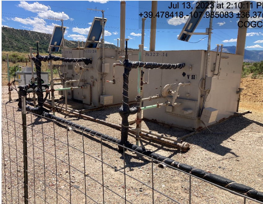
Separators and Meter calibration card not conspicuously posted.
