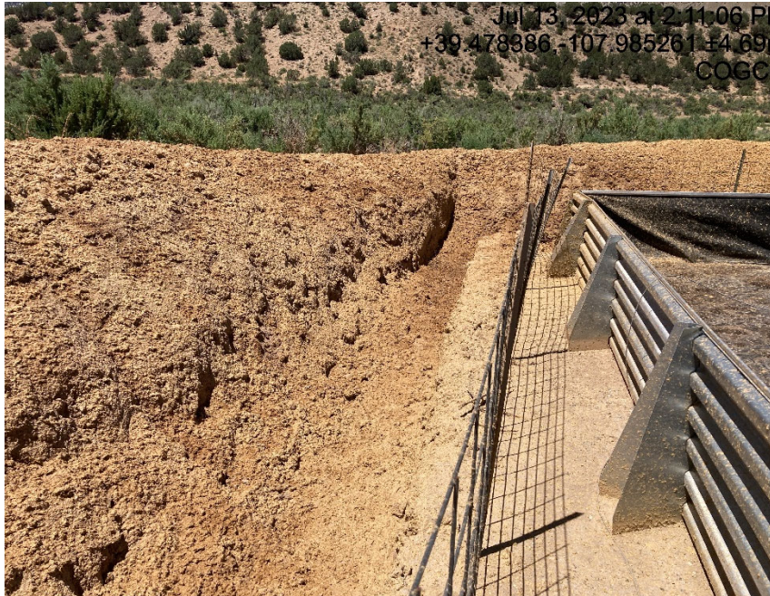
Hydro mulch on berms and ditch behind separators and tank battery
