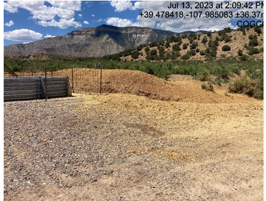
Hydro mulch on berms and ditch behind separators and tank battery
