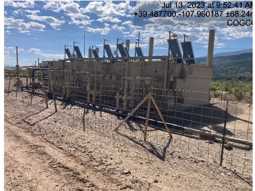
Separators and Meter calibration card not conspicuously posted.
