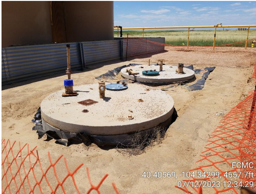
Photo 15 – Produced Water Vaults
