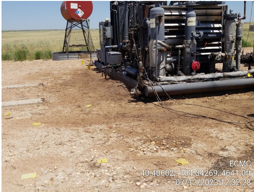
Photo 9 – Stained Soil Compressor and Locate Flags
