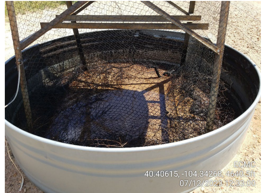
Photo 10 – Compressor Day Tank Wildlife Netting and Debris
