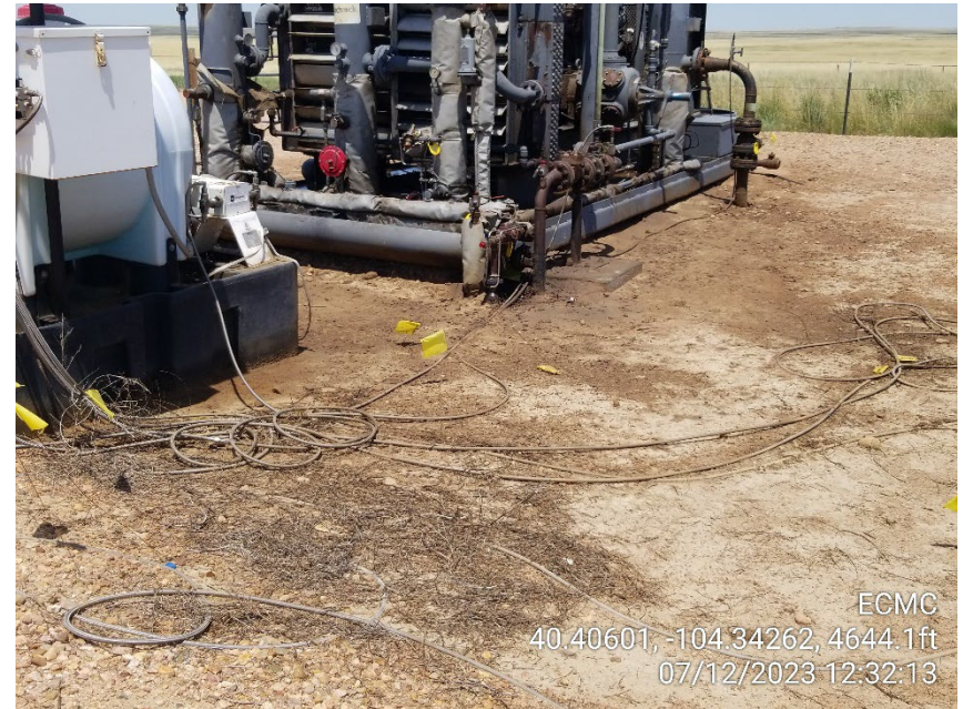
Photo 8 – Stained Soil at Compressor and Locate Flags
