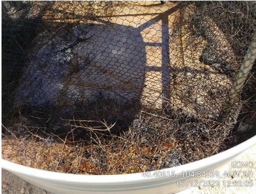
Photo 11 – Compressor Day Tank Wildlife Netting and Debris
