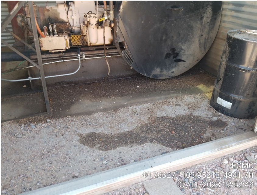
Photo 7 – 02-0214AH Stained Soil at Gas Engine
