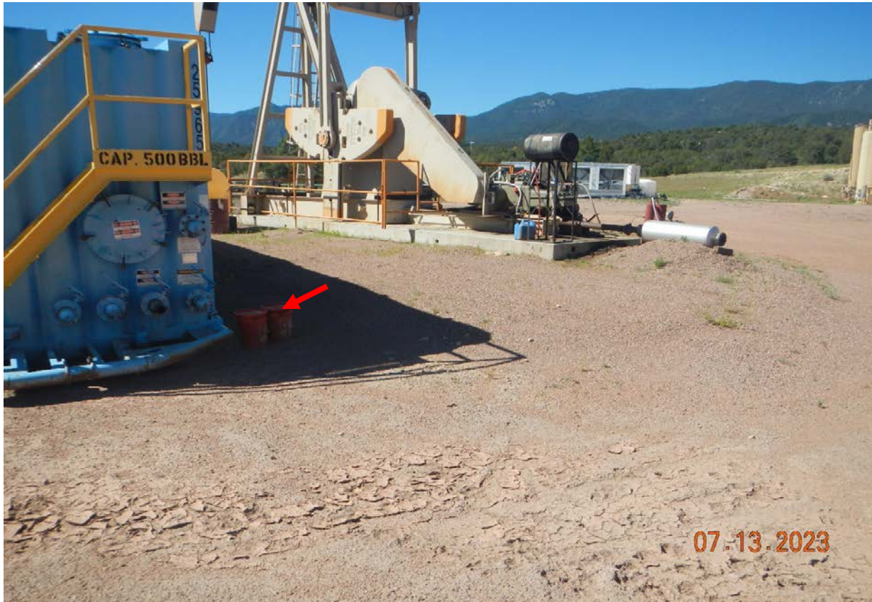
Photo 2. There are 2 orange buckets that appear to have oil with no labeling and no containment. Previous corrective action was not completed.
