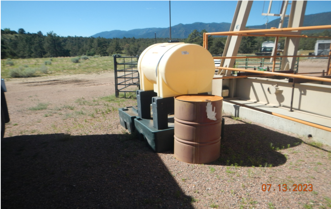
Photo 3. There is an unknown barrel with no labeling or containment. Previous corrective action was not completed.
