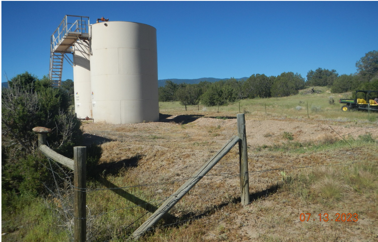
Photo 6. Facing southwest toward the tank battery. The fence around the tank is not maintained to prevent wildlife entry.
