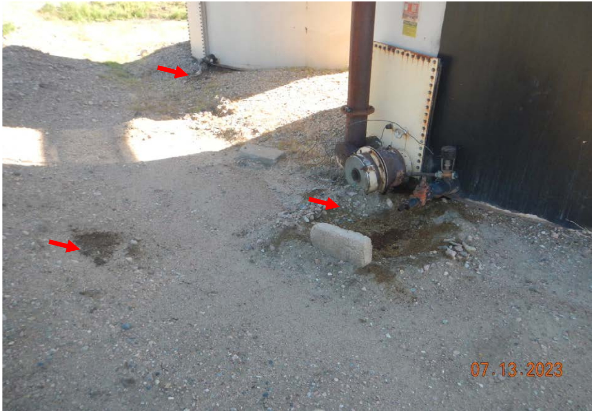
Photo 7. There is oil stained soils at back side of tanks shown at red arrows. Previous corrective action was not completed.
