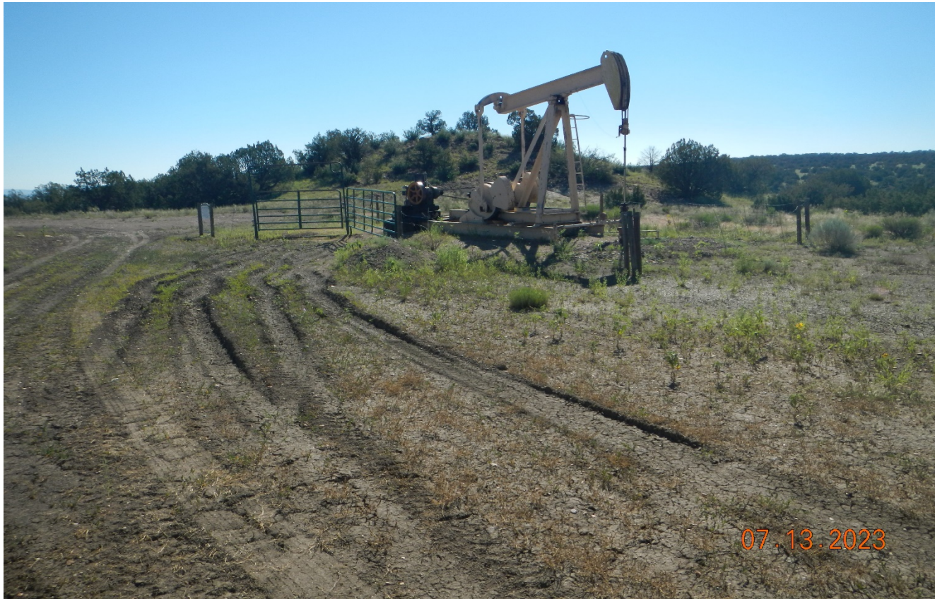
Photo 8. Facing northeast toward the wellsite. There is vehicle rutting at the location which is not stabilized. Previous corrective action was not completed.
