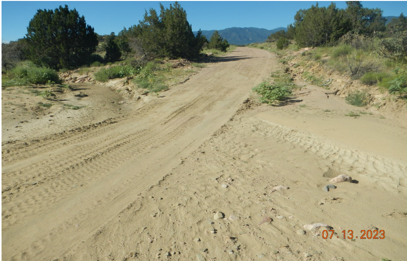
Photo 1. Facing south along the access road. There is erosion that occurred at the drainage crossing from recent storm event. The road has been washed out and needs to be repaired and BMP's need to be installed at the drainage crossing such as an adequately sized culvert. Previous corrective action was not completed.
