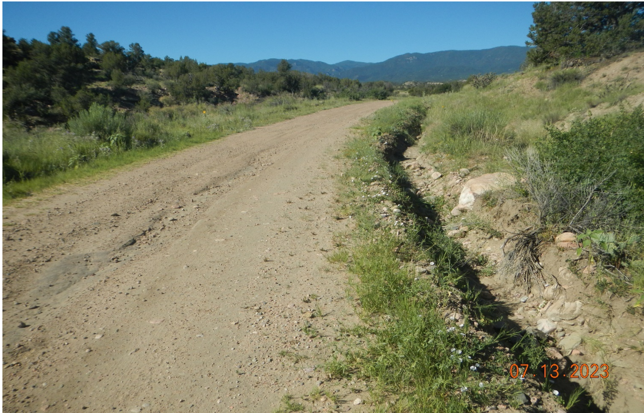
Photo 4. Further along the road is additional erosion on the road side that needs to be repaired and stabilized with BMP's. Previous corrective action was not completed.
