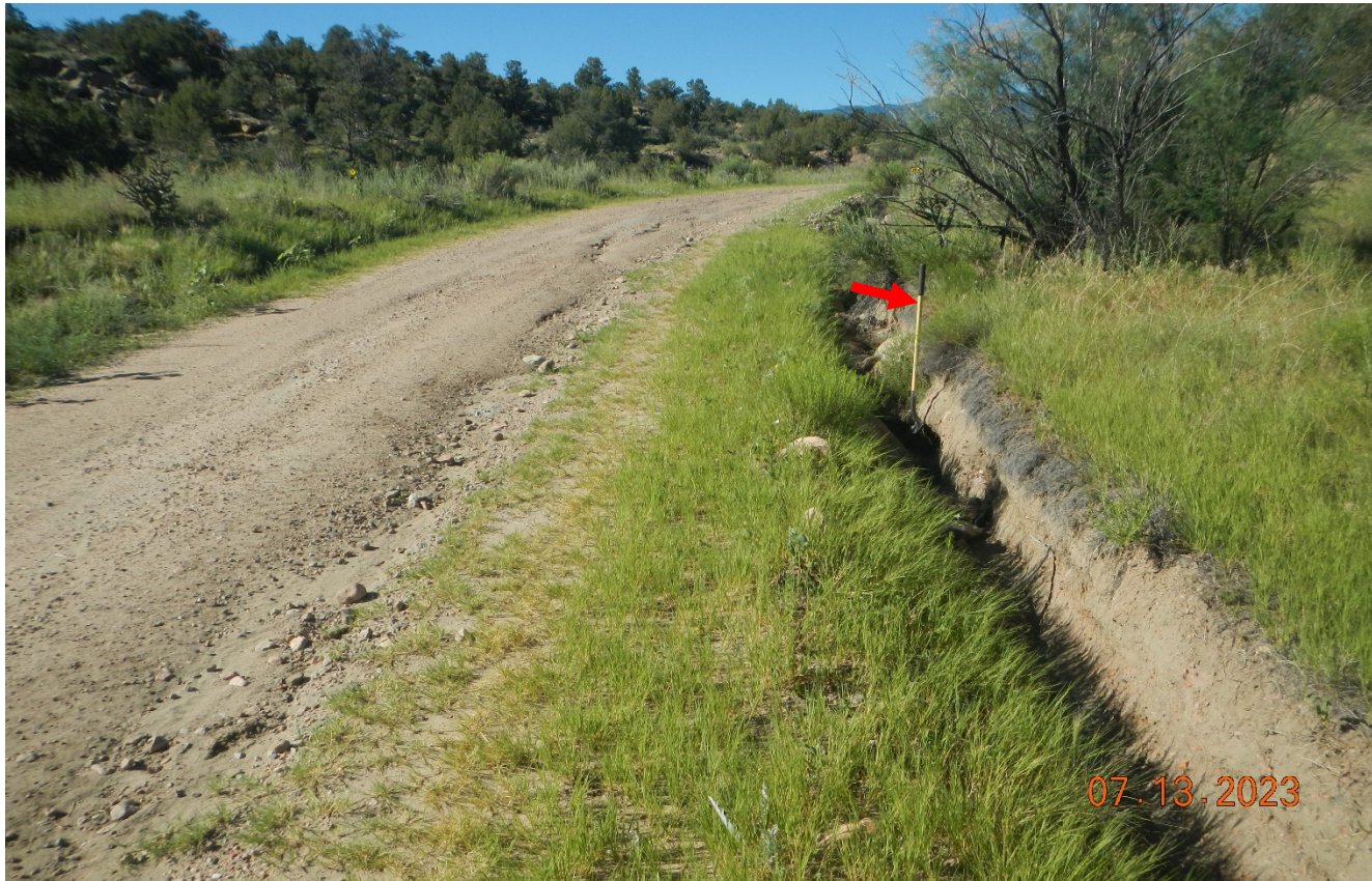
Photo 2. There is erosion along the road side that needs to be repaired and stabilized with BMP's. Red arrow points to 4.5' shovel for scale. There is a long stretch from this point further along the road with no culverts to divert stormwater off the road. Additional BMP's need to be installed along the road. Previous corrective action was not completed.
