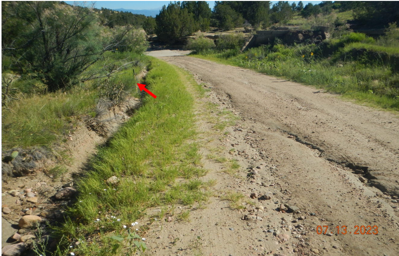
Photo 3. Facing back north at same area of erosion shown in previous photo. Stormwater and sediment is directed toward the creek drainage and needs to be repaired and stabilized to prevent erosion. Previous corrective action was not completed.
