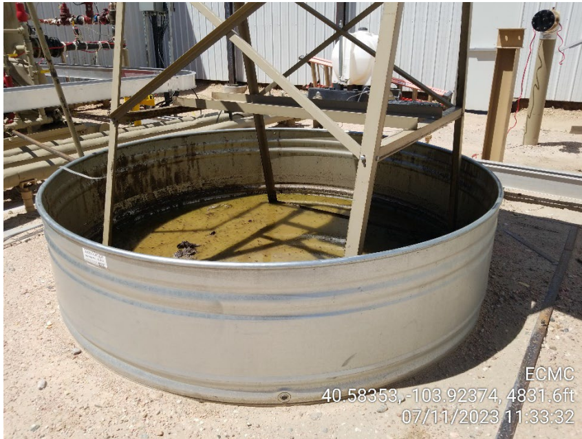
Photo 17 – Compressor Day Tank – Missing Wildlife Netting
