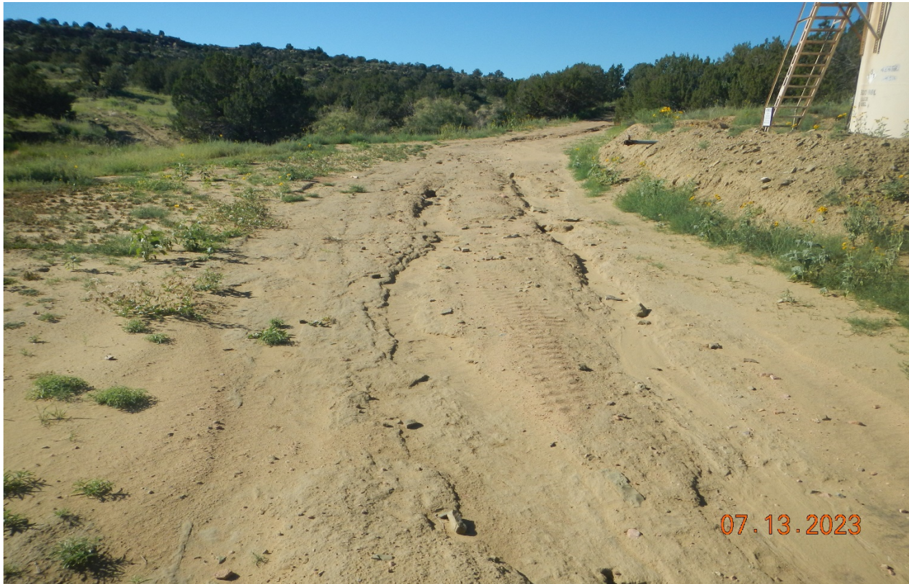
Photo 6. Facing southeast at the tank battery site. The equipment that was stoered along the east side of the road was removed. The disturbed area along the road side needs to be reclaimed and stabilized. There is erosion along the road that needs to be repaired and stabilized. Previous corrective action was not completed.
