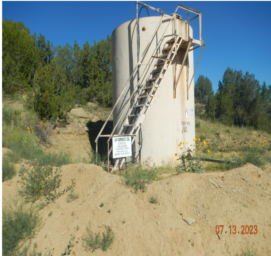
Photo 8. Facing toward the tank battery. The tank appears to be empty. There was a previous dripping leak observed at backside of the tank.
