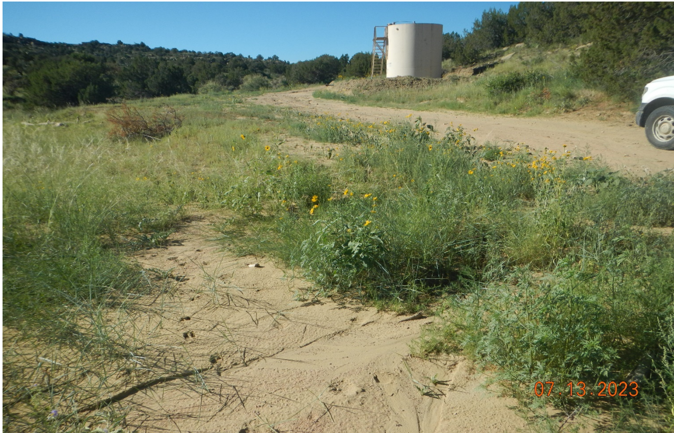
Photo 5. Facing southeast long the access road near the tank battery site. Recent storm event has washed sediment down the road and offsite into the stream drainage.
