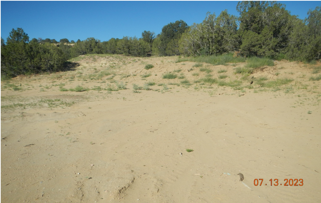
Photo 20. Facing southwest at the location. There are no stormwater run-on controls along the west side of the location. Recent storm event has caused erosion of the cut slope and stormwater was directed down the access road causing further erosion. Previous corrective action was not completed to install stormwater run-on controls.
