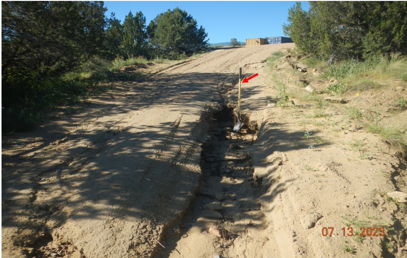
Photo 11. Facing south along the access road to the wellsite location. The road was never stabilized with BMP's and has continued to erode since previous inspection. Red arrow points to 4.5 ft. shovel for scale of erosion gully on the road.
