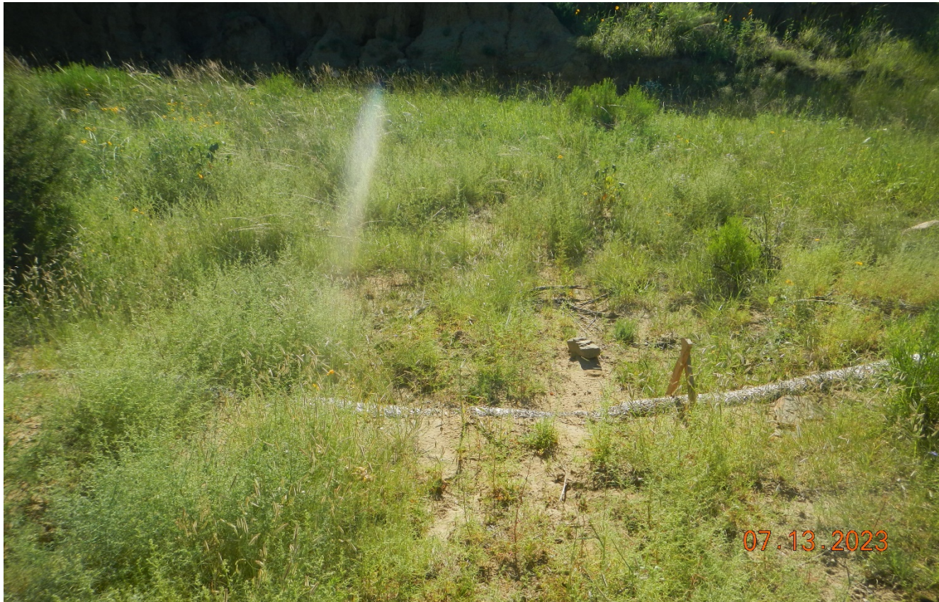
Photo 7. Facing southeast at the perimeter of the disturbance at the east side of tank battery. The wattles are not maintained and are filled in with sediment. corrective action was not completed.
