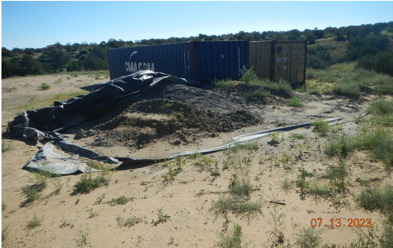
Photo 16. There is drill cuttings on the surface not properly stored and contained which is piled up behind the storage containers. The plastic liner does not contain the drill cutting and stormwater has transported the cutting off the liner toward the area shown in previous photos. Previous corrective action was not completed.
