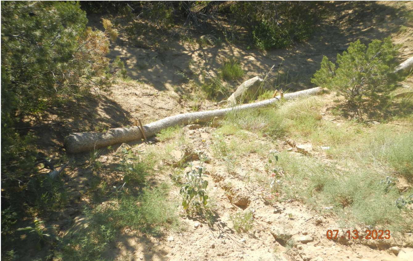
Photo 13. The wattles at the east perimeter were not properly installed and stormwater eroded underneath the wattles transporting sediment offsite. This issue still has not been fixed since previous inspection.
