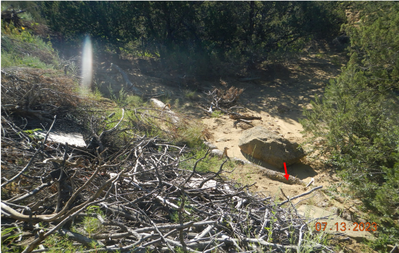
Photo 18. The wattles at the south side base of the fill slope have filled in with sediment and are not maintained. The wood debris dumped along the side of the fill slope has not been removed. Previous corrective action was not completed.
