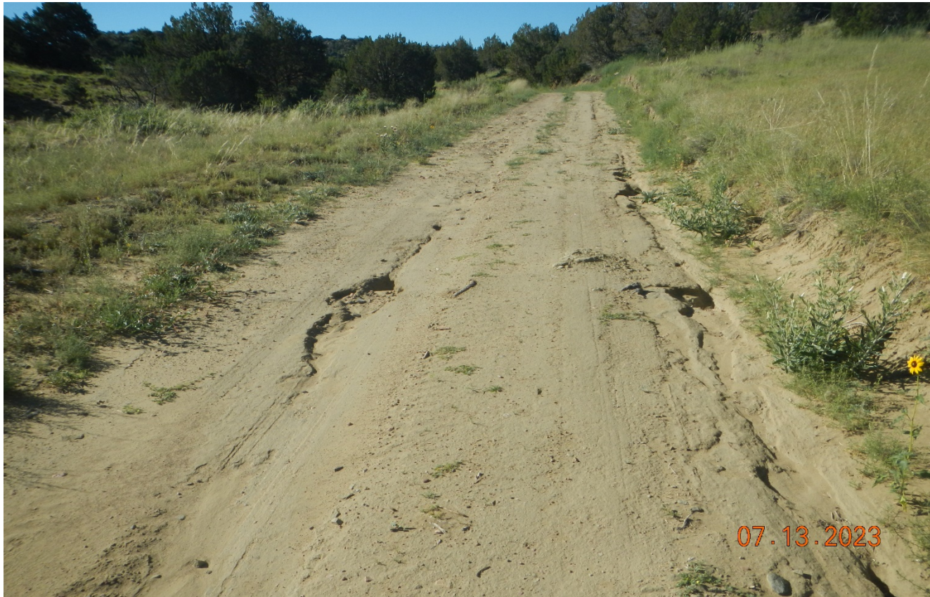
Photo 4. Facing southeast long the access road. There is erosion along the access road which is not stabilized and no BMP's have been installed. Previous corrective action was not completed.
