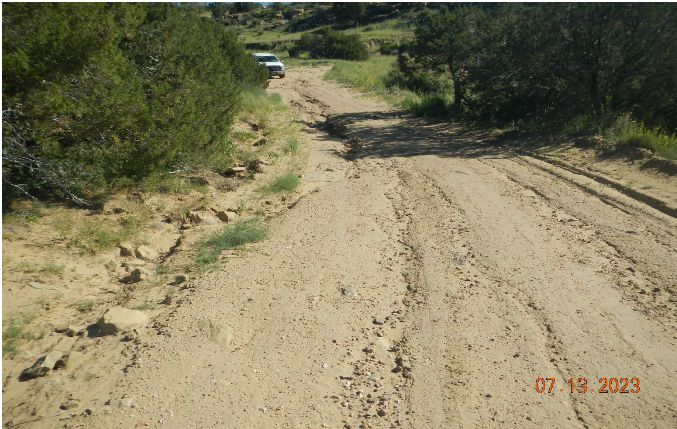
Photo 21. Facing back to the northeast toward the access road. Stormwater directed from the location shown in previous photo caused erosion of the access road which transported sediment off site.
