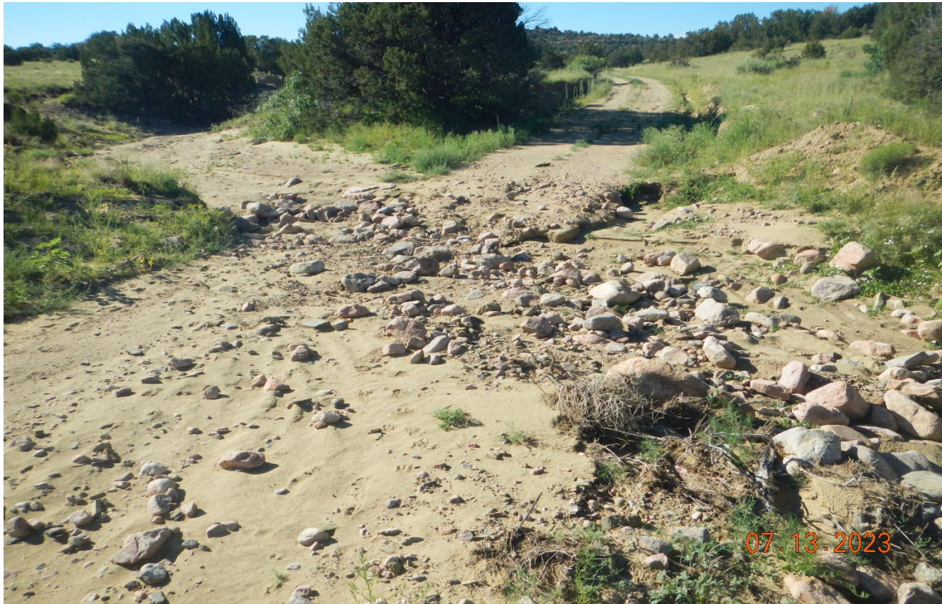
Photo 2. Facing southeast long the access road. This drainage crossing must have BMP's installed to accommodate seasonal storm event to prevent material from washing out. BMP may include culvert, rip/rap, ect. Previous corrective action not completed. Storm events have caused further erosion of the road since previous inspection.
