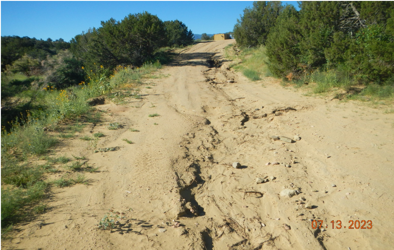
Photo 10. Facing south along the access road to the wellsite location. The road was never stabilized with BMP's and has continued to erode since previous inspection. .
