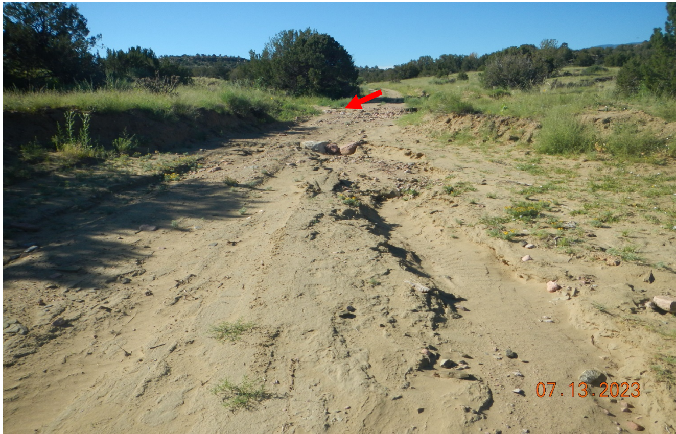
Photo 1. Facing southeast long the access road. Erosion has occurred from a recent storm event which washed down from the drainage at red arrow. Previous corrective action required culvert or other BMP to be placed at the drainage which may have prevent erosion of the road. Previous corrective action was not completed.
