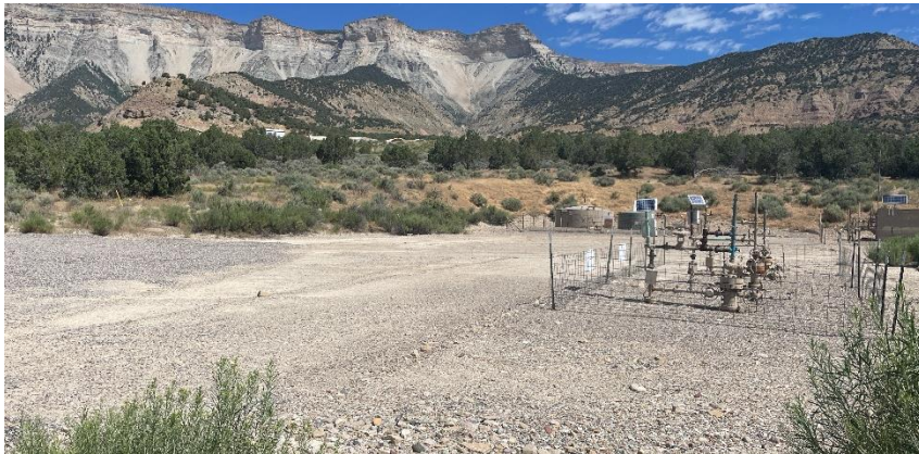
South West corner of location.
