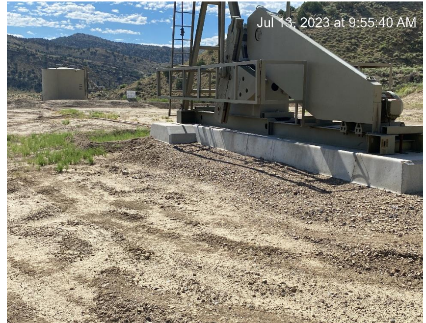
Location from Northwest corner
