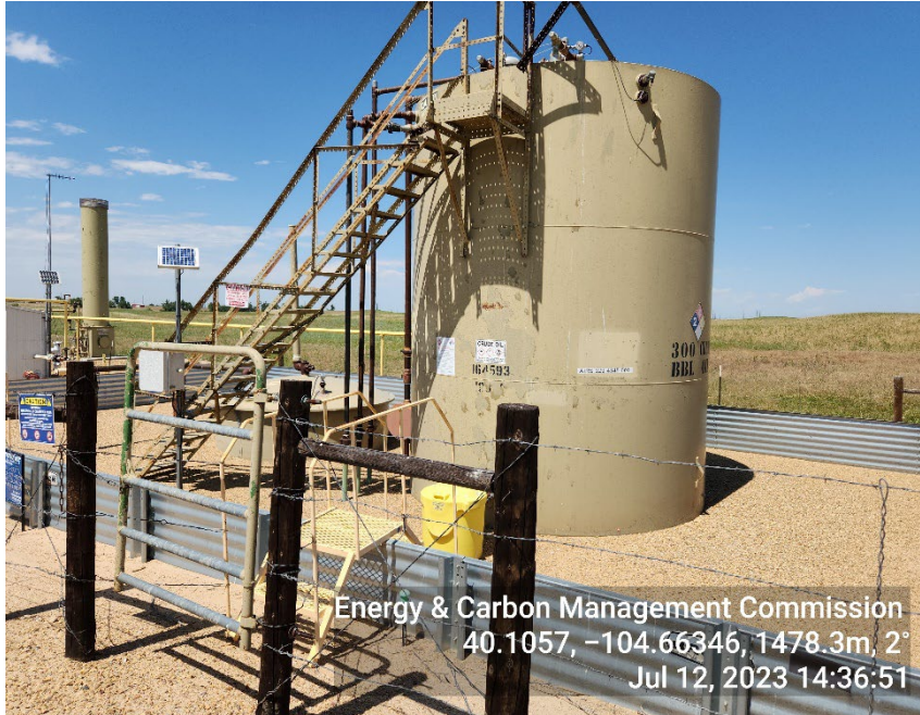
Photo 3: Tank Battery
