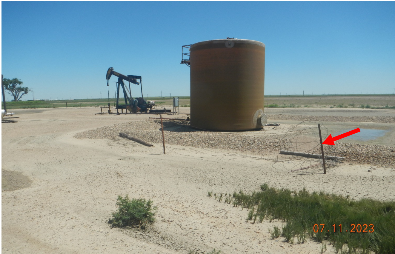
Photo 1. Facing southeast toward the wellsite. The fence at the tank battery is in disrepair shown at red arrow.
