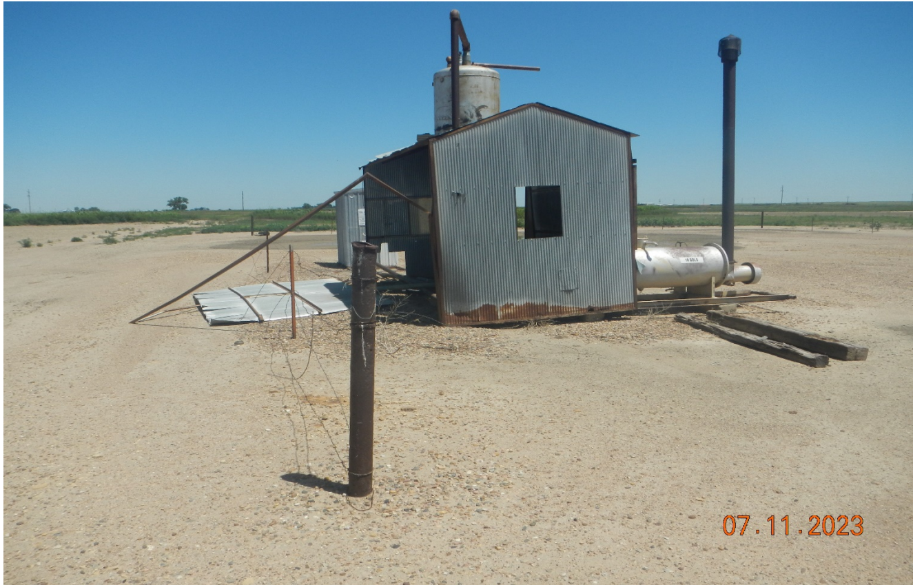
Photo 2. Facing east toward the separator shed. The fence at the shed is in disrepair and the shed wall is laying on the ground.
