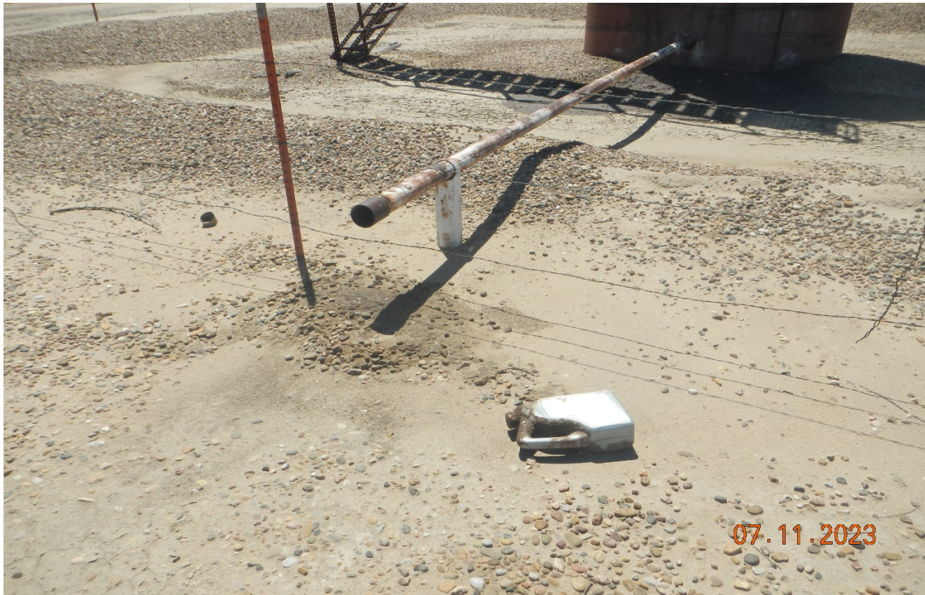
Photo 3. There is oil stained soils at the tank pipe outlet. There is a plastic oil container that needs to be removed and disposed.
