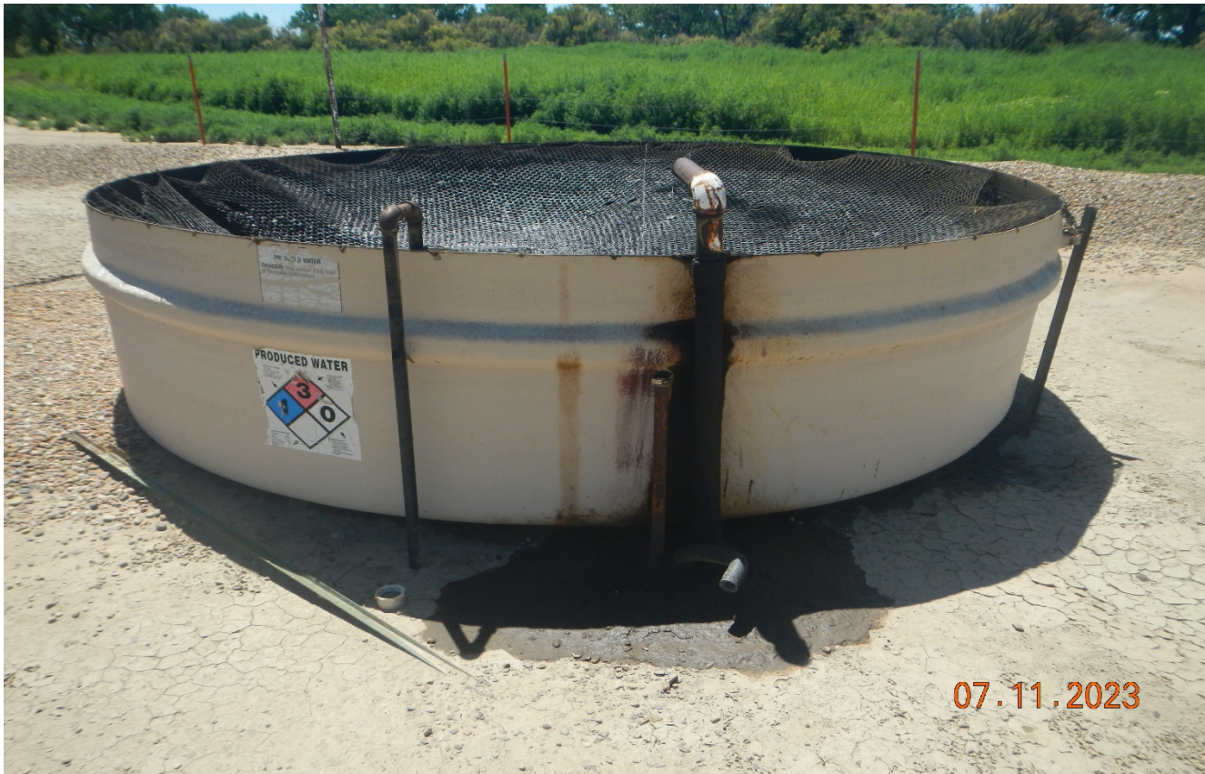
Photo 5. There is oil staining that overtopped the open top tank. There is oil inside the tank and the tank is mislabeled as produced water.
