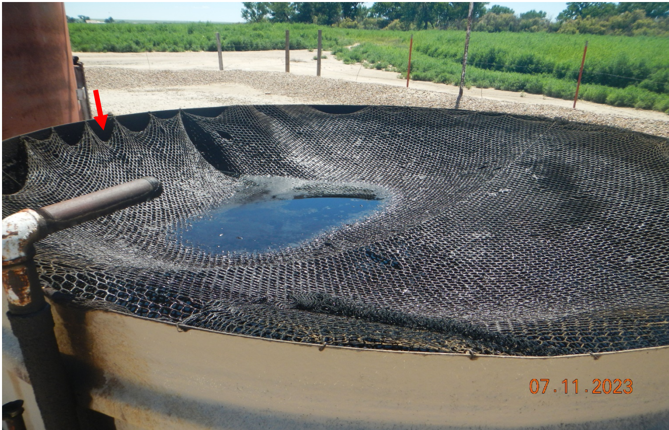
Photo 6. The netting on the open top tank is insufficient to prevent wildlife entry. There are openings at red arrow and oil level is over the netting.
