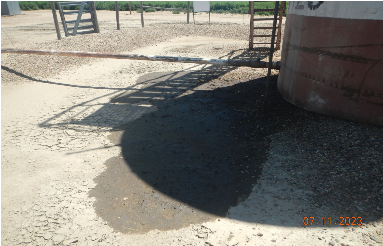
Photo 4. There is oil stained soil at the tank that needs to be cleaned up. It appears to have leaked out from the tank but no leak was observed at time of inspection.
