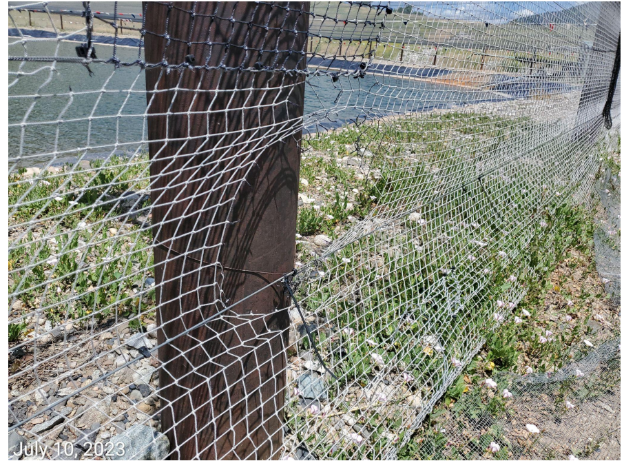
Photo 6: Photos examples showing holes observed in netting at pits.
