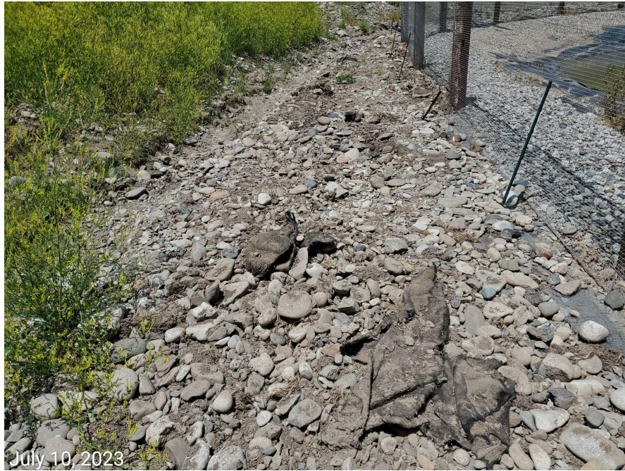
Photo 3: Liner material in disrepair. Material is now considered debris.
