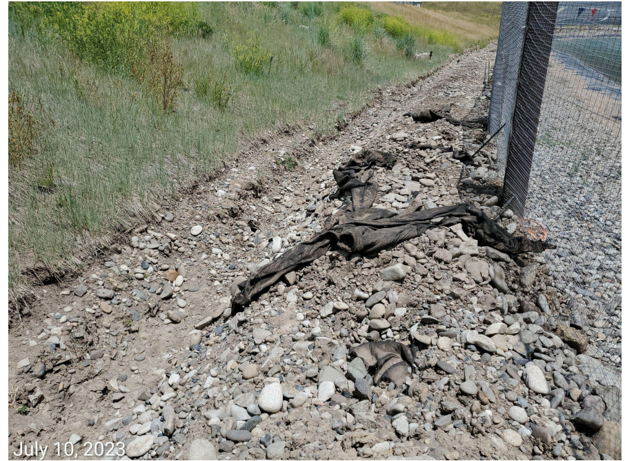
Photo 3: Liner material in disrepair. Material is now considered debris.
