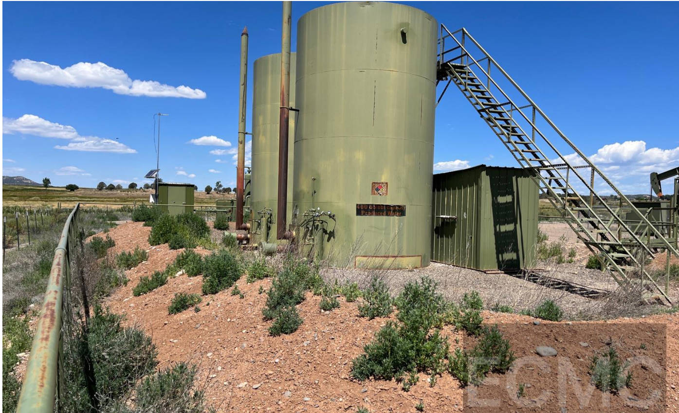
Photo #3. View of weeds growing on tank containment berm.
