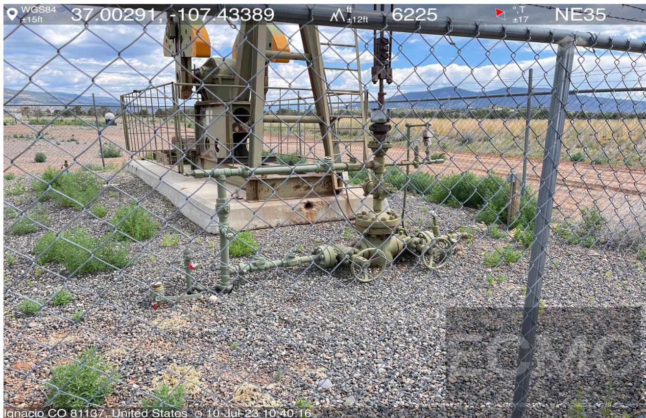
Photo #2. View of the 19-2 wellhead assembly.
