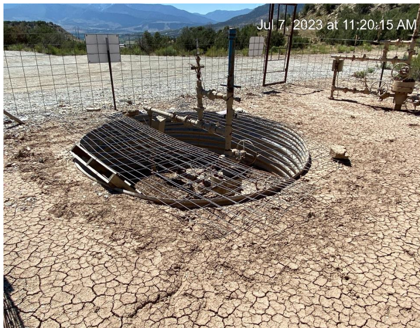
Cellar cover installed as a result of corrective action noted on last inspection
