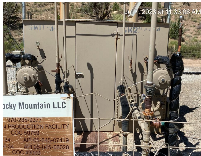
No visible display of gas meter calibration
