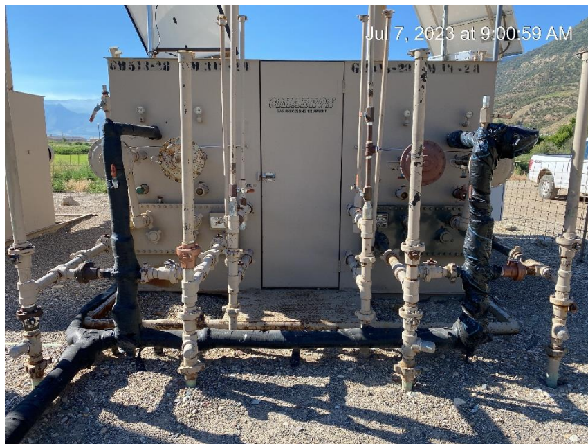
No visible display of gas meter calibration
