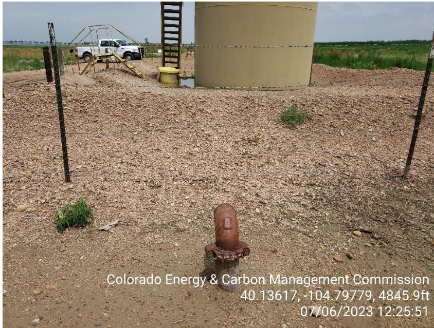
Photo 7 Unmarked, uncapped flow line not LOTO.
