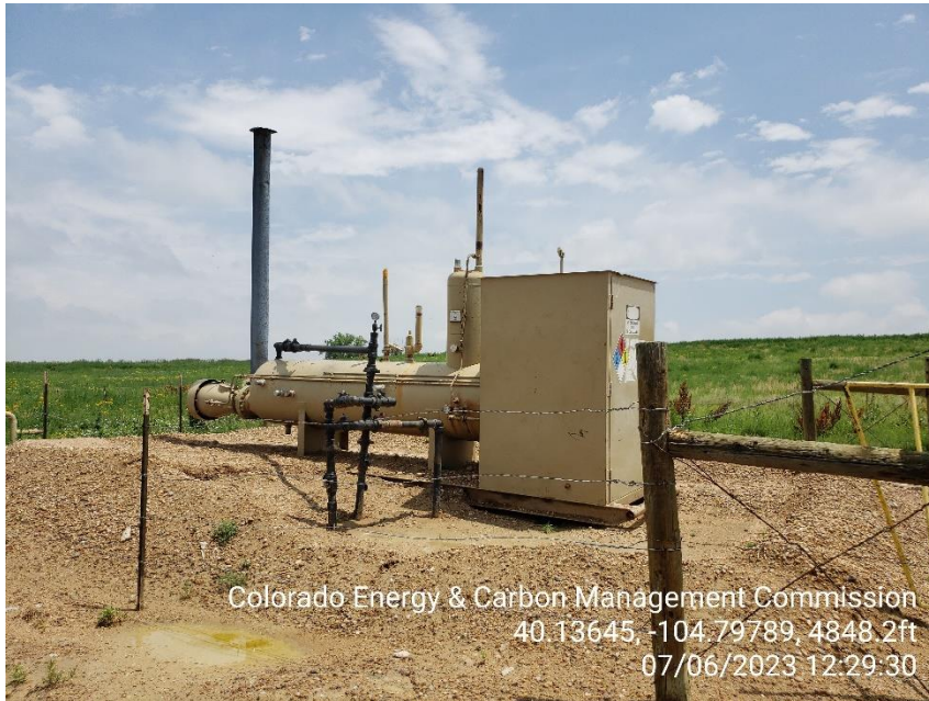
Photo 9 Horizontal Heated Separator.
