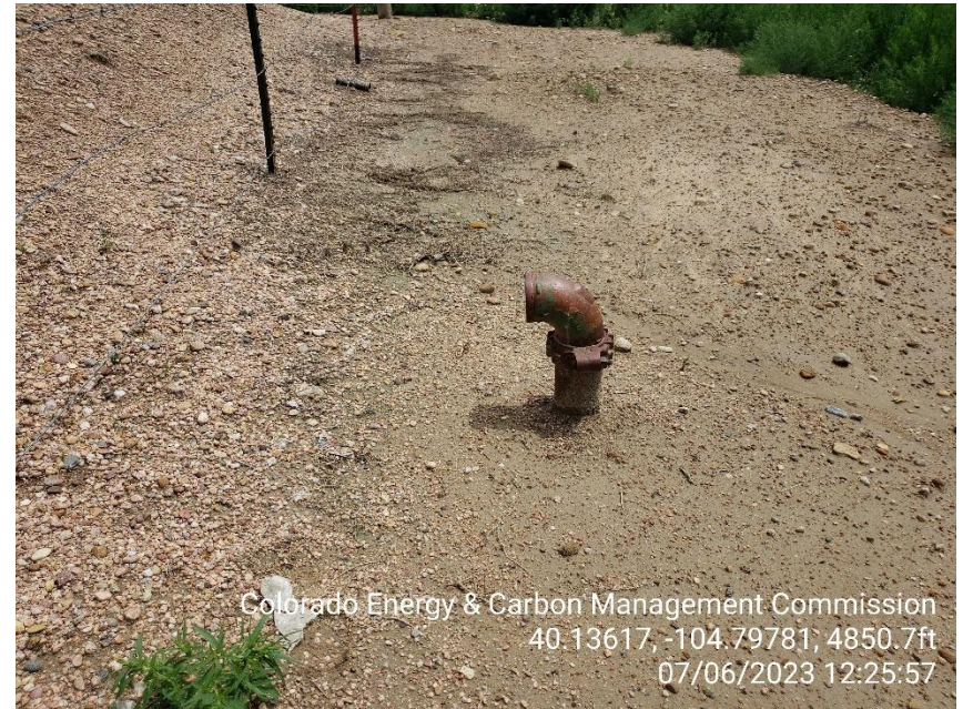
Photo 8 Unmarked, uncapped flow line not LOTO.
