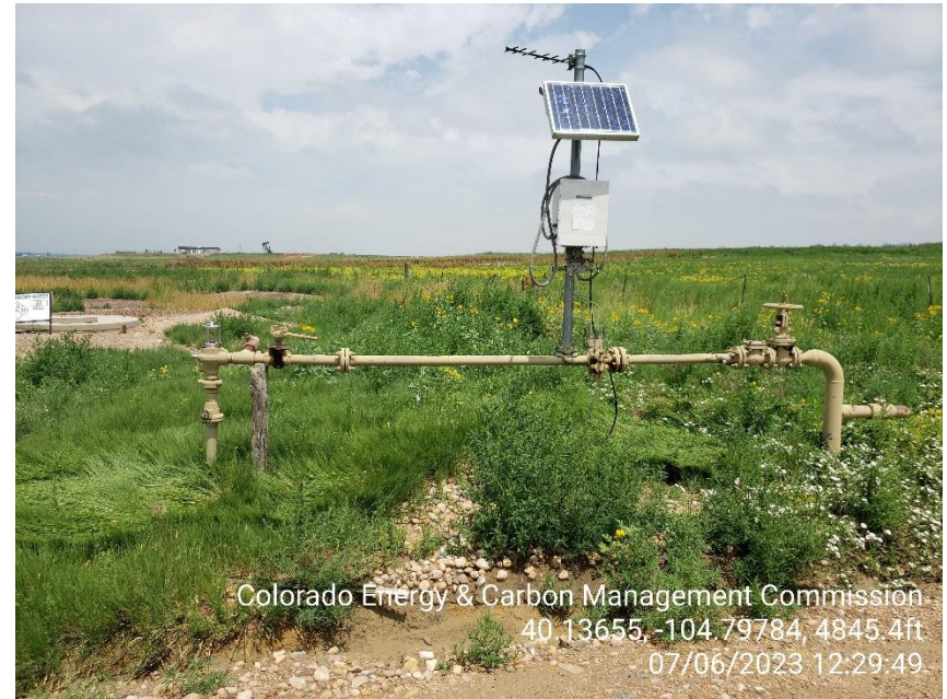
Photo 10 Gas Meter Run, no indication of calibration status.
