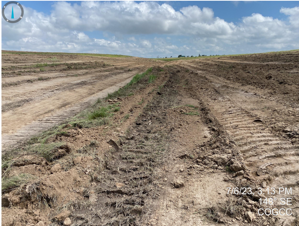
Photo 13. Taken from the center portion of the location; photo illustrates grubbing activities occurring within the fill areas.
