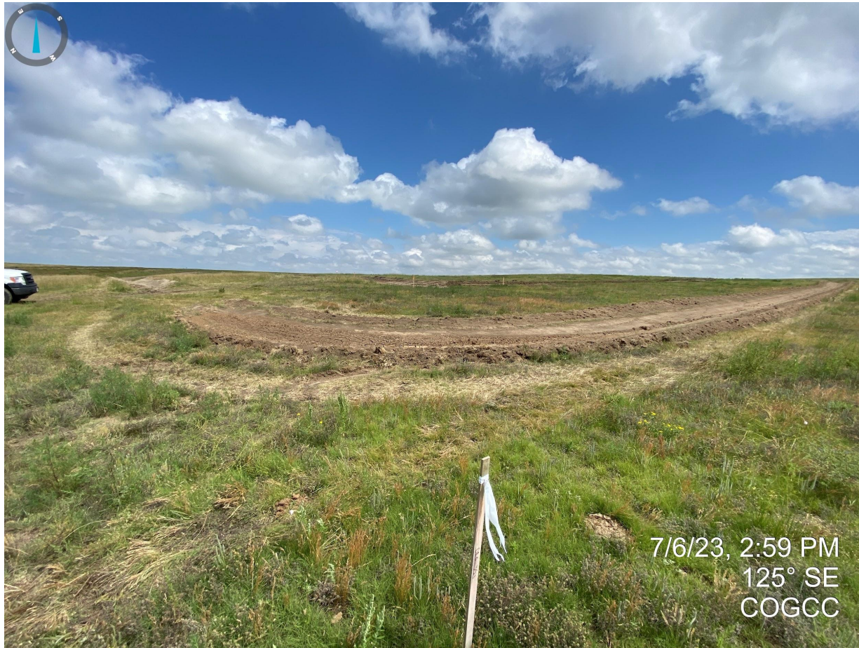
Photo 5. Taken from the northwest corner of the disturbance area. Photo illustrates that a perimeter ditch and berm has been constructed around the entire location.
