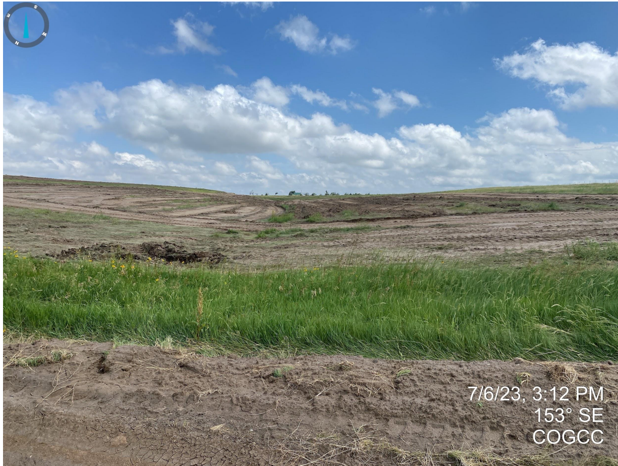
Photo 11. Taken from the northern, central portion of the location. It appears that grubbing activities have recently occurred. The Operator shall ensure that all topsoil has been separated and stored in accordance with Rule 1002.b. A follow-up inspection will be performed at a later date to verify compliance with topsoil salvage operations.
