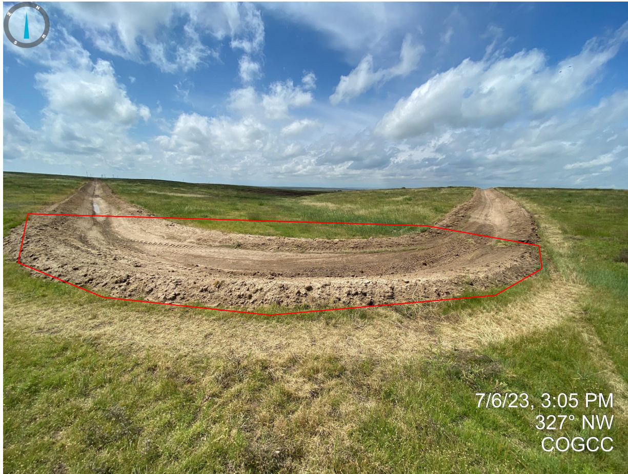
Photo 7. Taken from the southeast corner. Berm material does not appear to be properly stabilized with evidence of unconsolidated material.
