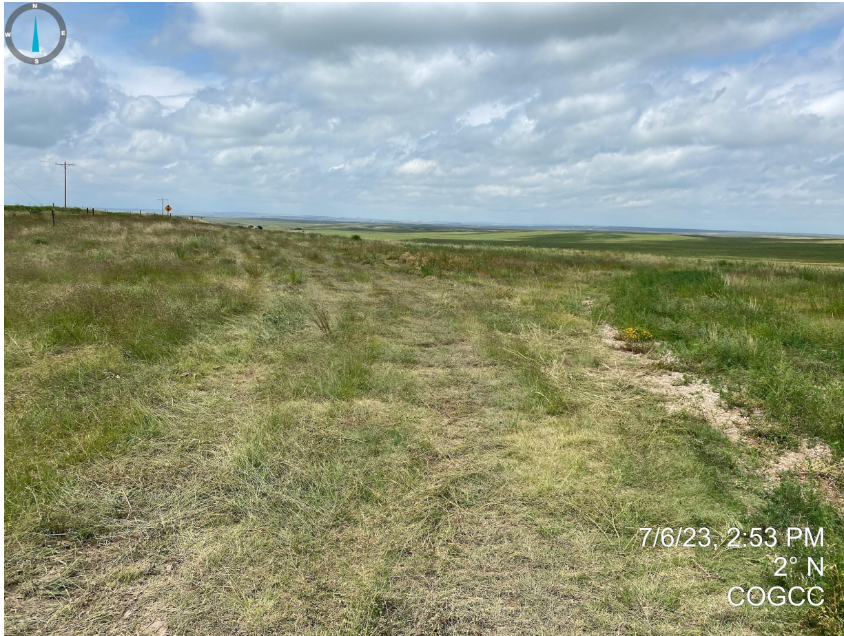
Photo 2. Facing north near the location entrance. Topsoil salvage has not occurred on the new access road; this will need to be completed per Rule 1002.b.
