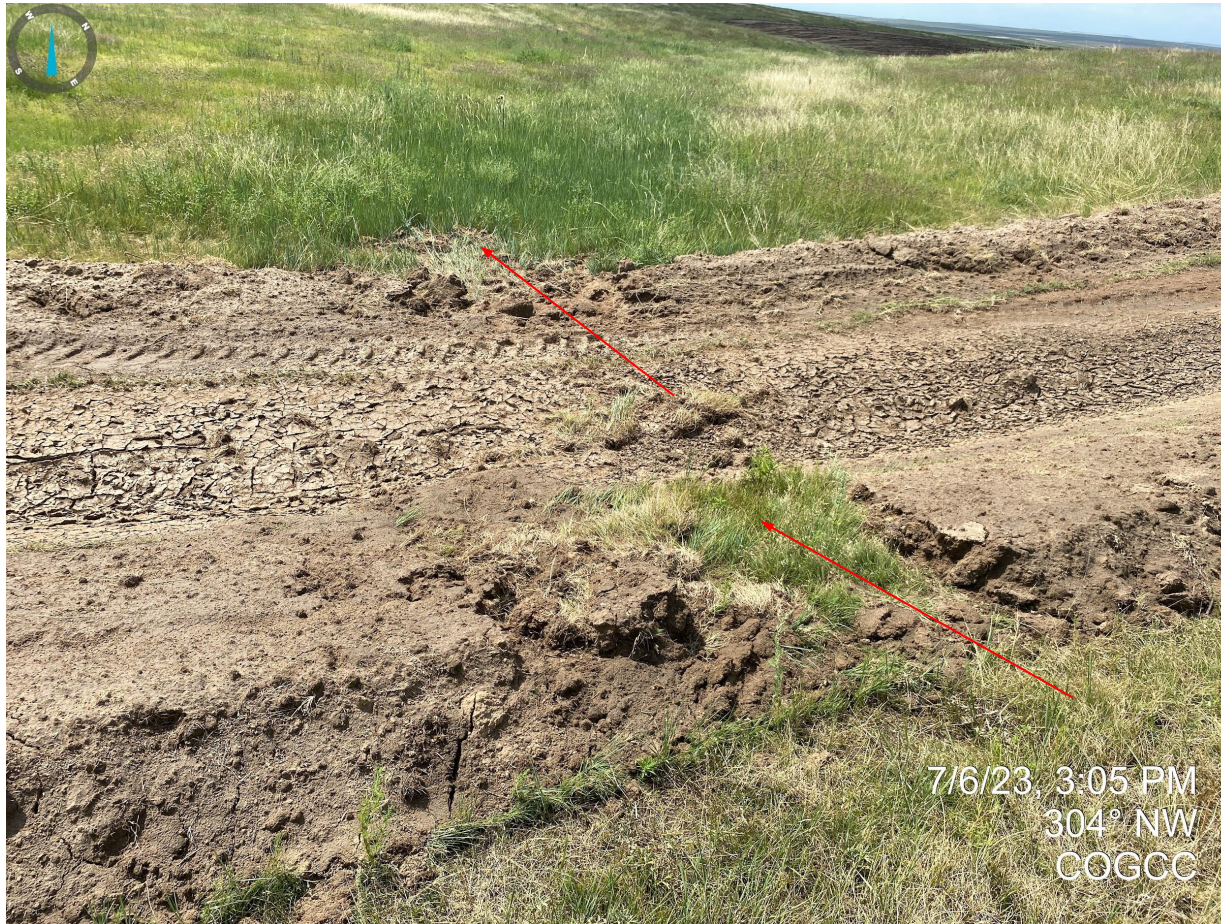
Photo 8. Taken near the southeast corner of the location. The berm material does not appear to be properly stabilized with evidence of unconsolidated material. It appears stormwater run-on has eroded a portion of the berm; additional maintenance or implementation of more robust BMPs is required.
