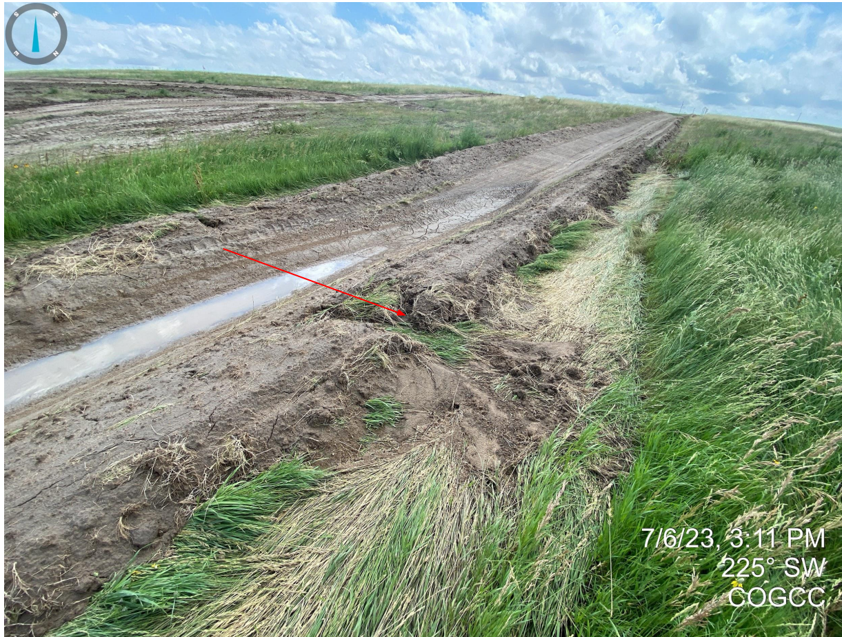
Photo 10. Taken from the northern, central, portion of the stormwater ditch and berm. The berm material does not appear to be properly stabilized with evidence of unconsolidated material. It appears stormwater runoff has eroded a portion of the berm; additional maintenance or implementation of more robust BMPs is required.
