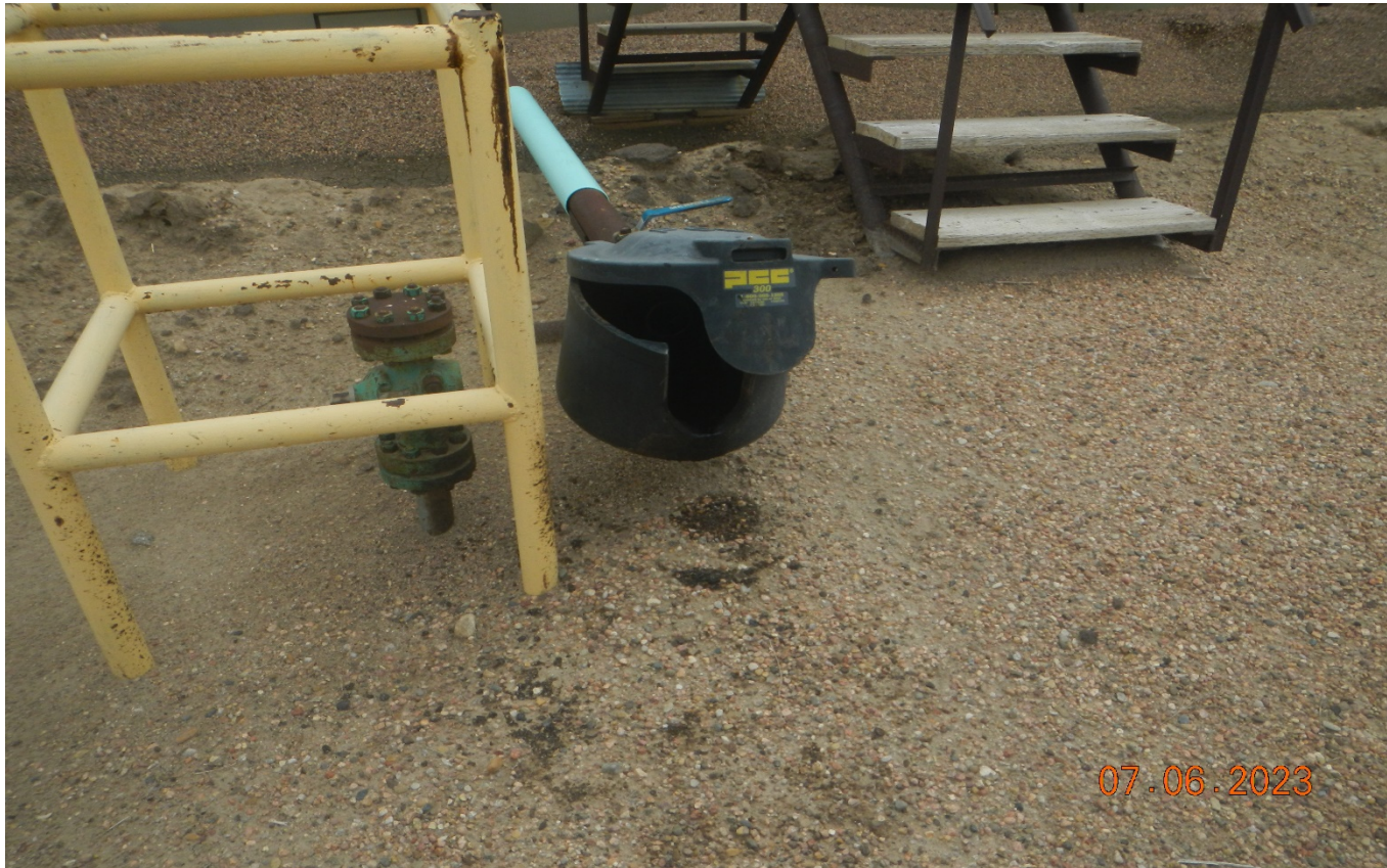
Photo 4. Facing toward the PYLES offsite tank battery at the location. There is still stained soil at the outlet and oil fluid inside the plastic containment.
