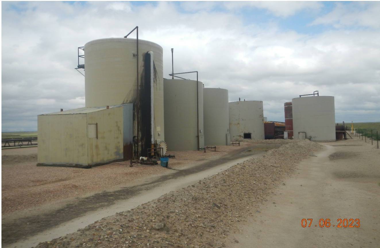
Photo 6. Facing at the back side of the tank battery. There was a spill from the tank which needs to be cleaned up. The blue bucket needs to be emptied and disposed of any oil.
