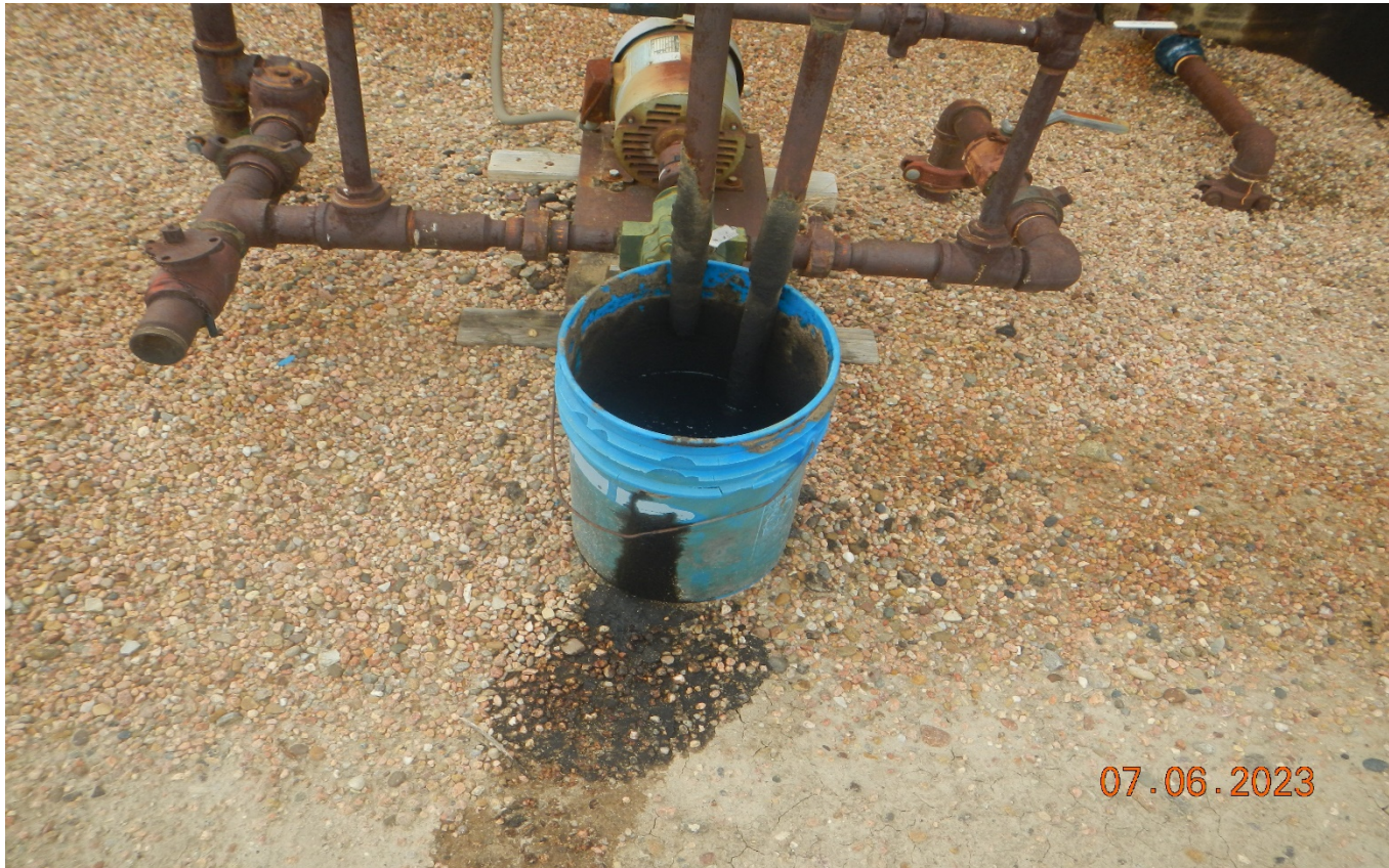
Photo 7. This bucket t the backside of the tank battery is full of oil which has spilled onto the ground.
