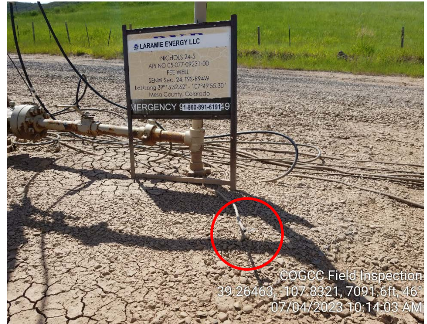
Photo #8 – Uncapped production pipe located at Nichols 24-5 wellhead.
