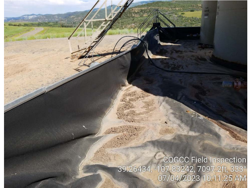
Photo #4 – View into tank battery secondary containment area.
