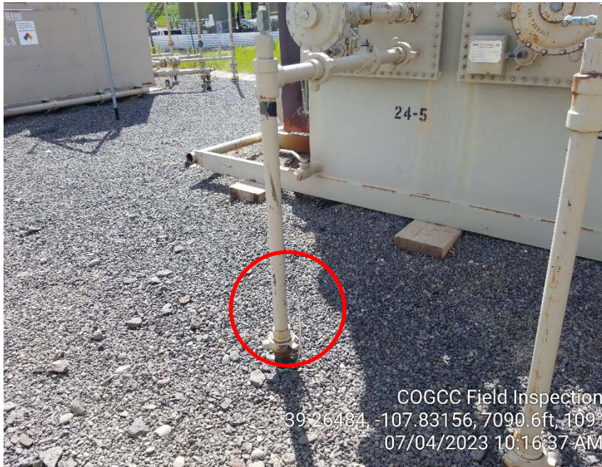
Photo #11 - Uncapped production pipe located at Nichols 24-5 separator.
