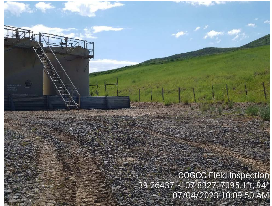
Photo #2 - Tire ruts at entrance to pad.
