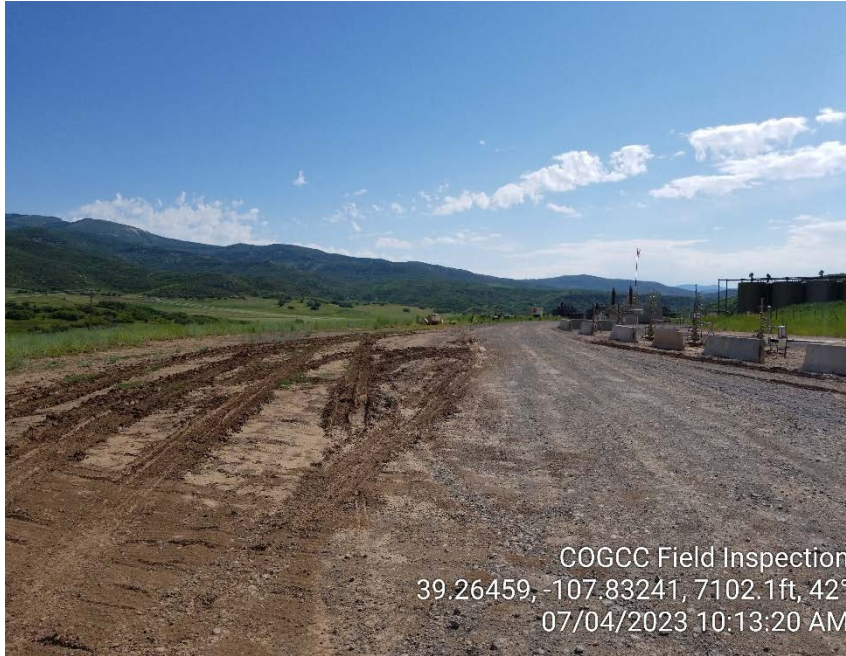
Photo #5 – Rutted area along NW side of pad.
