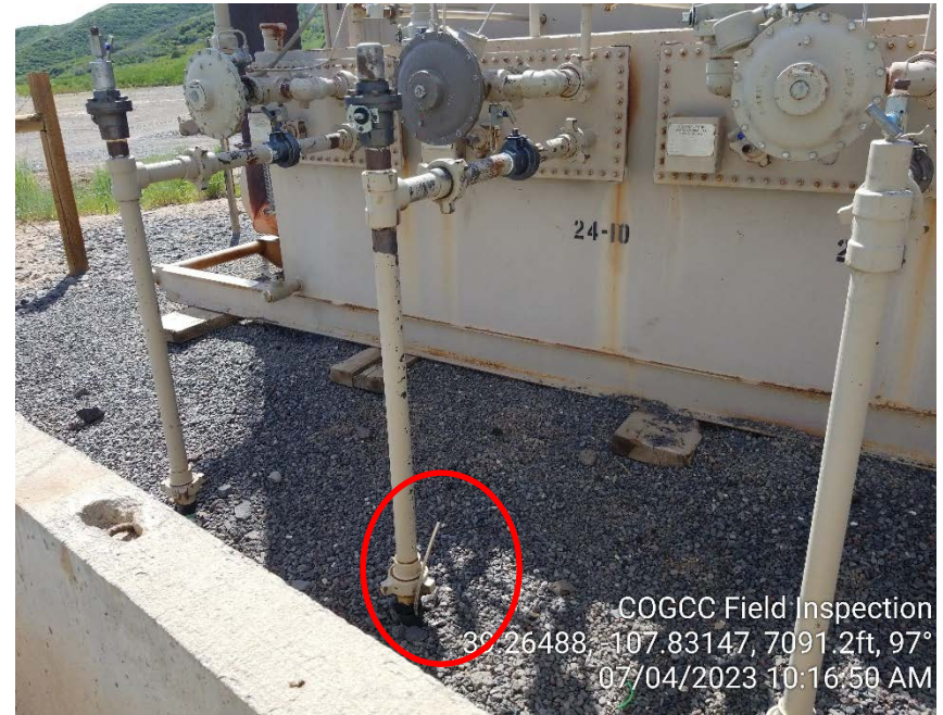
Photo #12 - Uncapped production pipe located at Nichols 24-10 separator.
