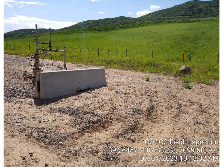
Photo #6 – Rutted area SW of wellheads.
