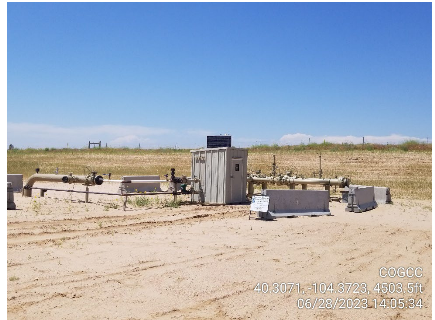
Photo 4 – Gas Meter and Pig Station
