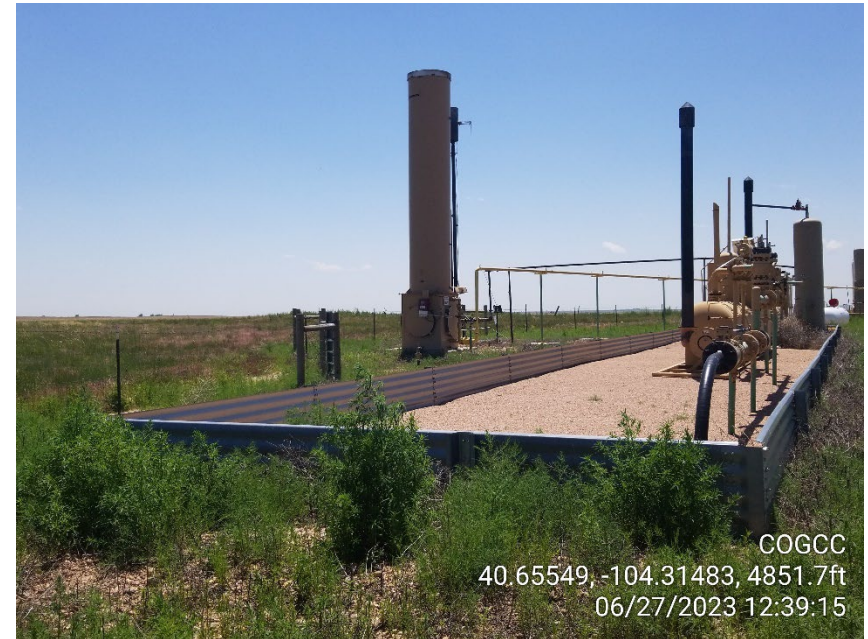
Photo 6 – ECD and Separator – WEEDS
