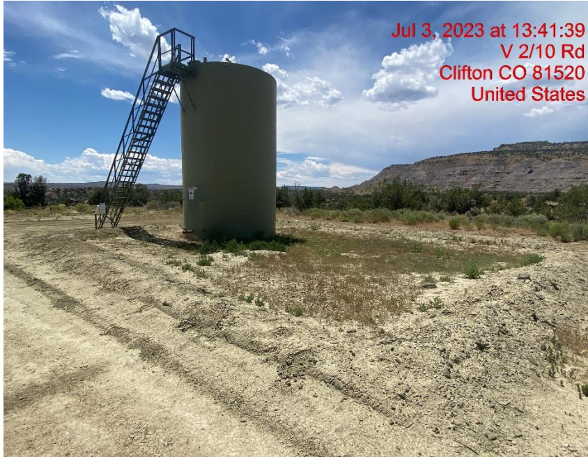
Tank Battery/Insufficient Capacity & Permeability of Secondary Containment – Photo #04992
