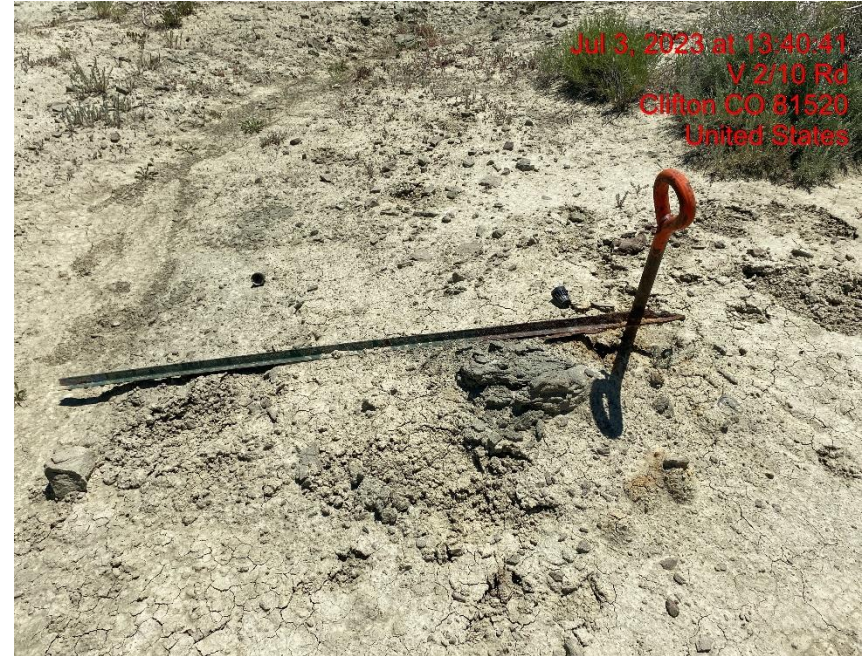
Anchor Not Properly Marked – Photo #04987
