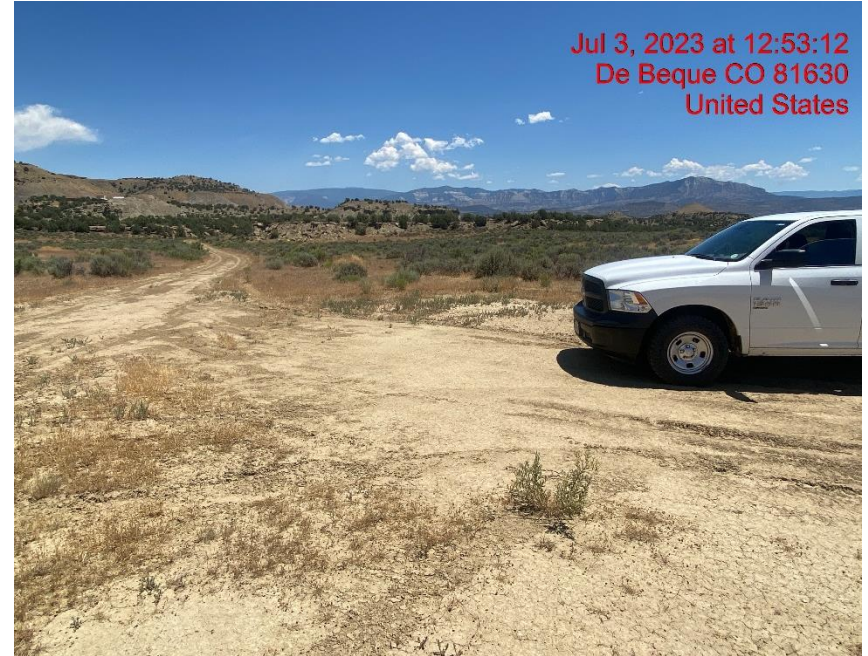
Insufficient Vehicle Tracking BMPs at Location Entrance/Exit – Photo #04961
