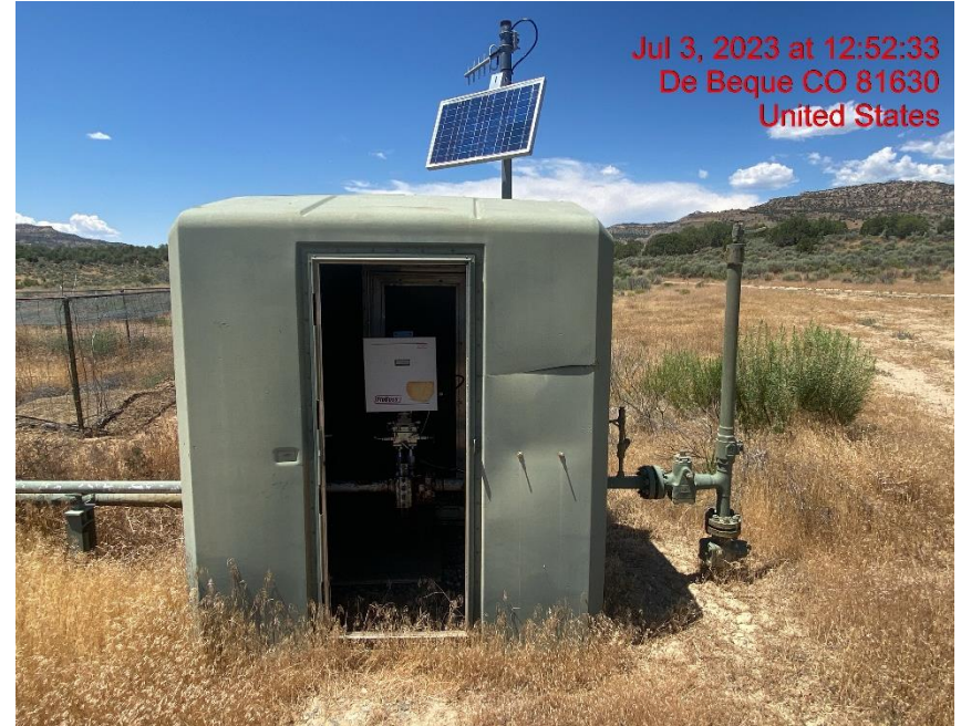
Unsecured Gas Meter/Weeds – Photo #04958
