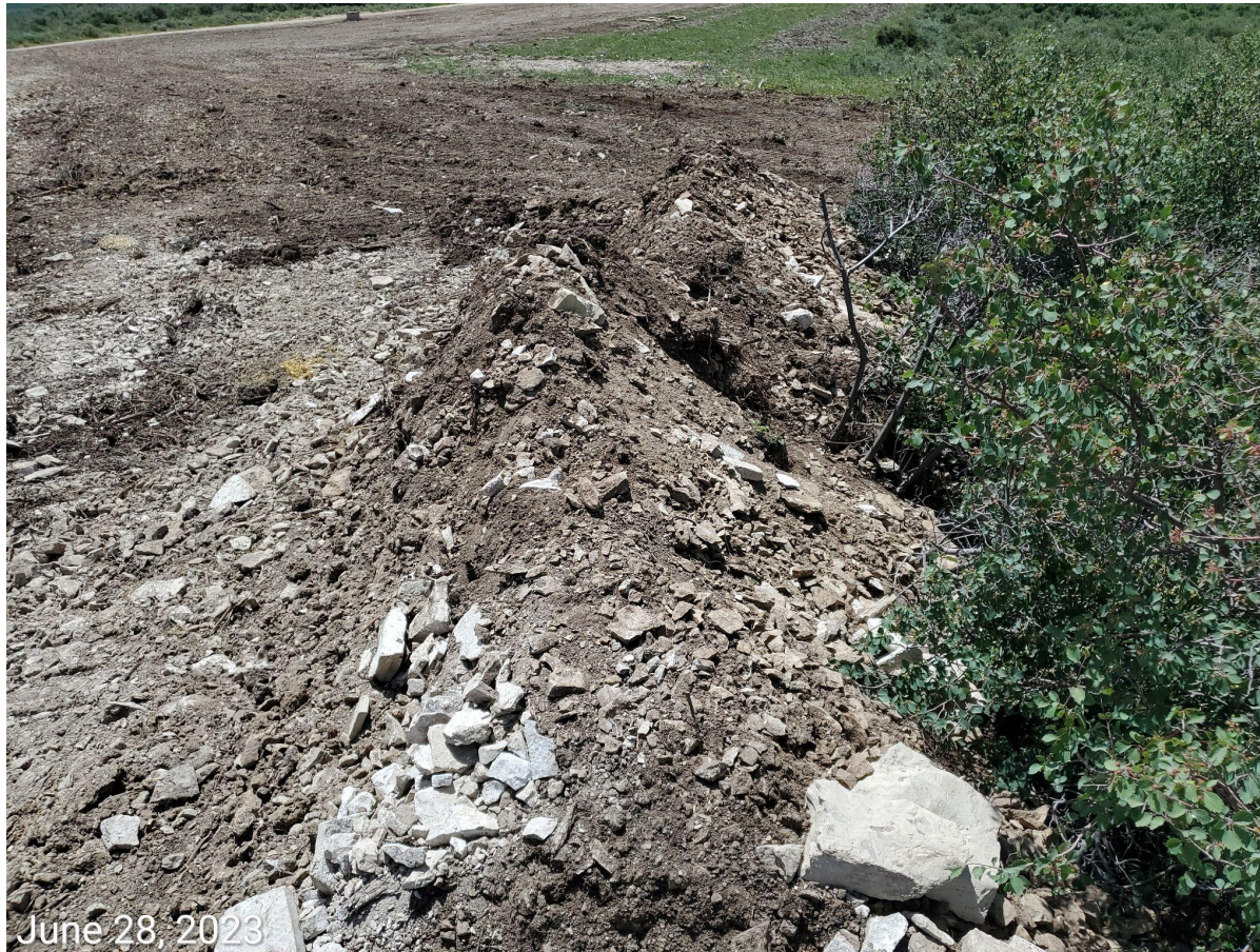
Photo 7: Photo taken from the south end of the Location. Photo shows BMPs to properly protect the topsoil, including BMPs to minimize erosion, degradation and sediment transport are missing or insufficient. Photo also show Operator appears to have mixed subsoils with the topsoil.
