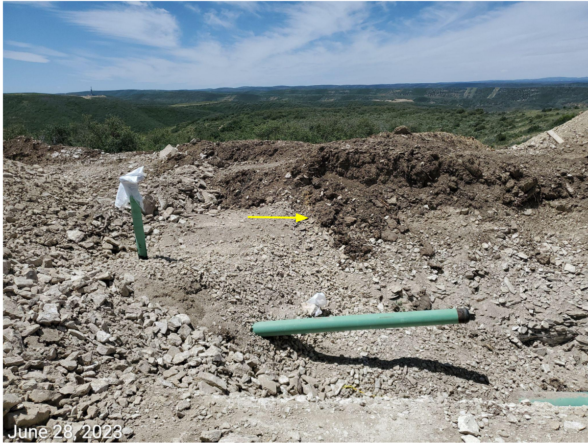
Photo 6: Photo taken from the south end of the Location. Photo shows topsoil eroding into the excavation. BMPs to properly segregate and protect the topsoil are missing or insufficient.
