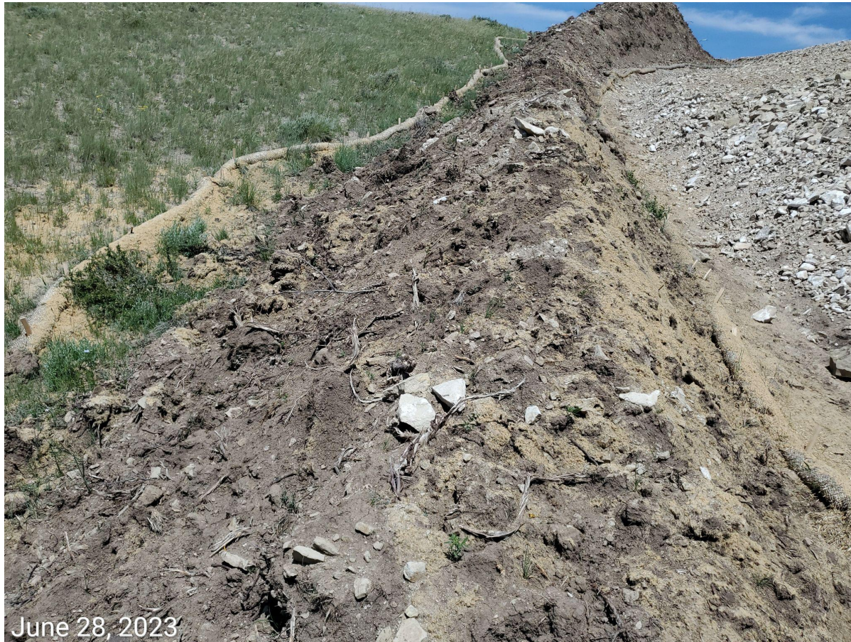
Photo 11: Photo taken from the topsoil stockpile on the west end of the Location. This photo is an example showing Operator had applied hydromulch to the soil stockpiles and slopes throughout the Location. Hydromulch only appears to have been applied to the east facing slopes, and/or has degraded throughout the majority of the areas where it has been applied; BMP is no longer in proper functioning condition to protect/stabilize the soil stockpiles/slopes.
