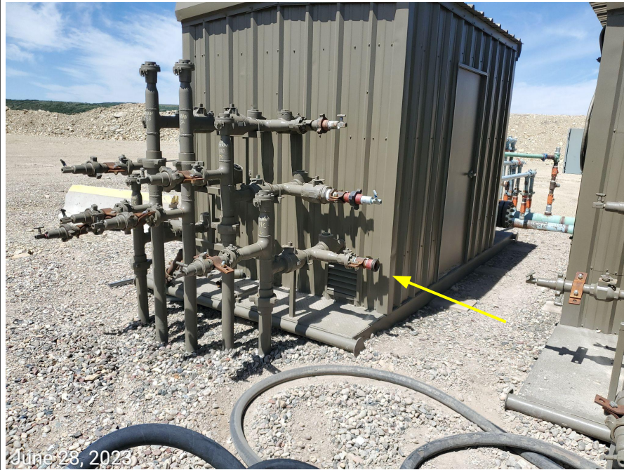
Photo 15: Photos 15-16 examples showing lines/pipe at and around the separator equipment not properly capped.
