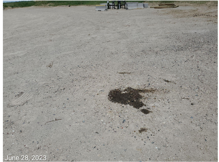
Photo 5: Stained soils at separator equipment and north end of the Location.
