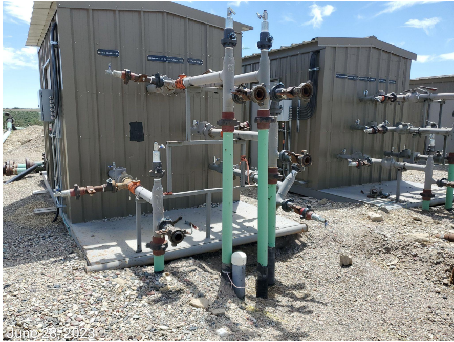
Photo 6: Photos examples showing pipes/lines at separator equipment not properly capped.
