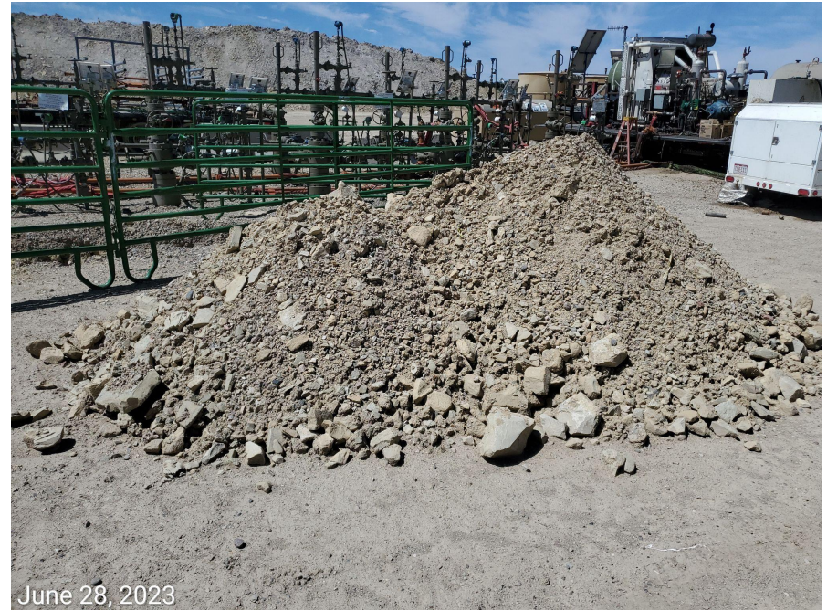
Photo 10: Soil stockpiles on Location missing BMPs per 1002.c
