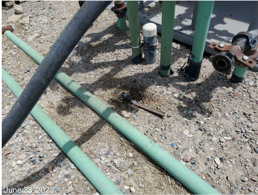
Photo 5: Stained soils at separator equipment and north end of the Location.
