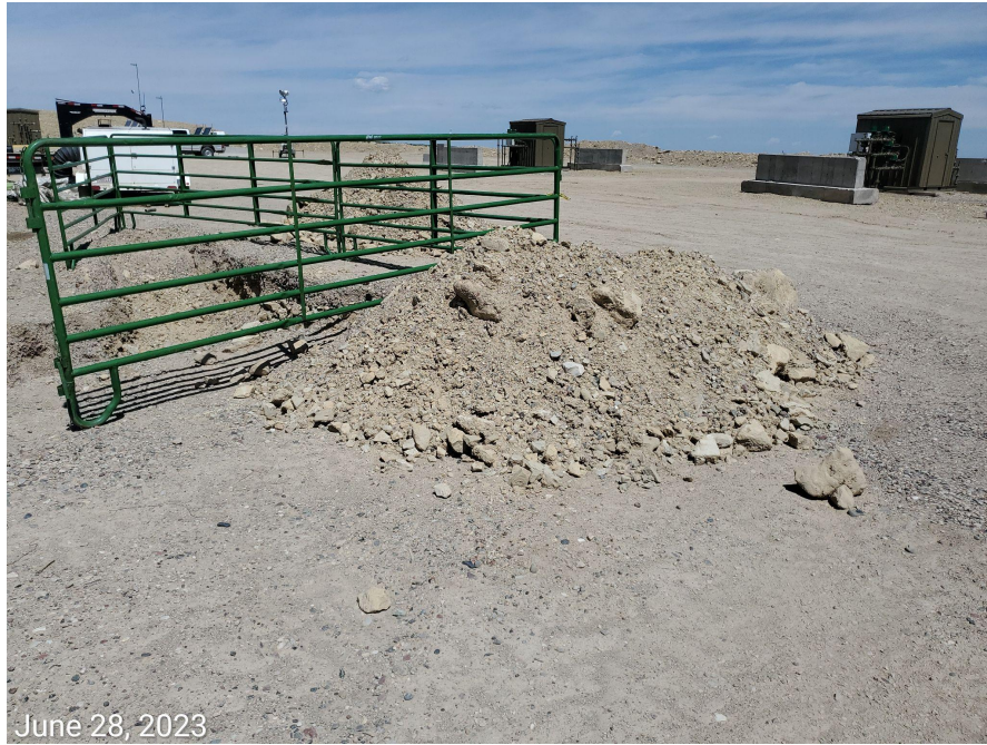
Photo 10: Soil stockpiles on Location missing BMPs per 1002.c
