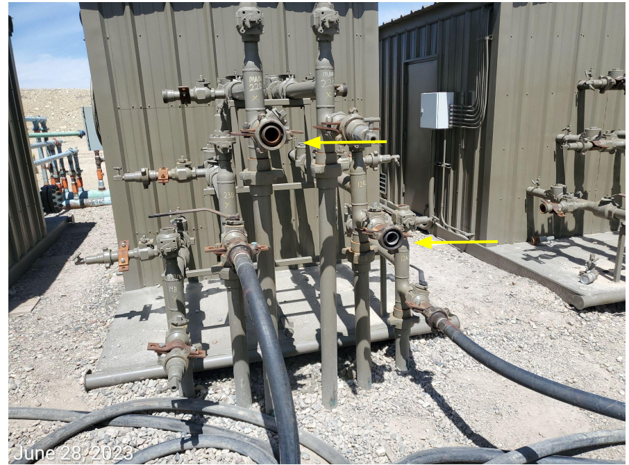
Photo 15: Photos 15-16 examples showing lines/pipe at and around the separator equipment not properly capped.
