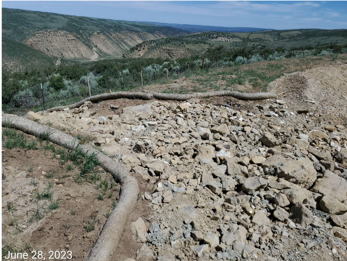
Photo 18: Sediment trap and outlet on west end of the Location.
