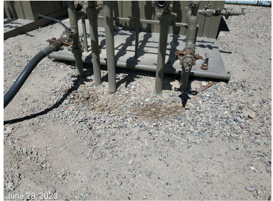
Photo 13: Stained soils around battery and separator equipment.
