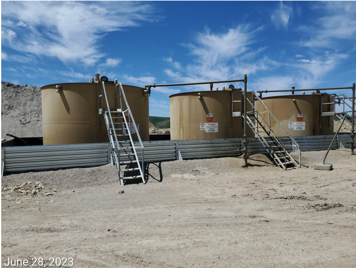
Photo 9: Tank battery facility missing required signage.
