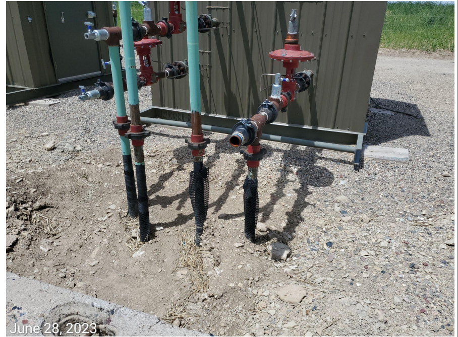
Photo 6: Photos examples showing pipes/lines at separator equipment not properly capped.
