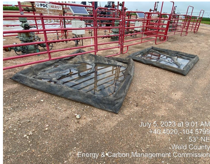
Unused Secondary containment
