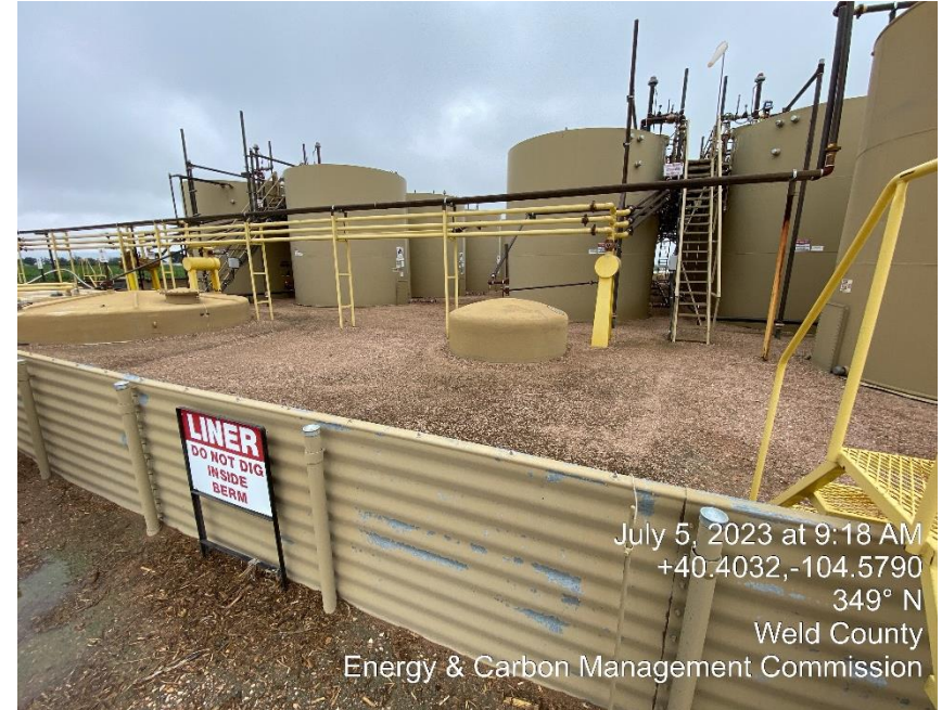
Missing signage/placard for small fiberglass tank
