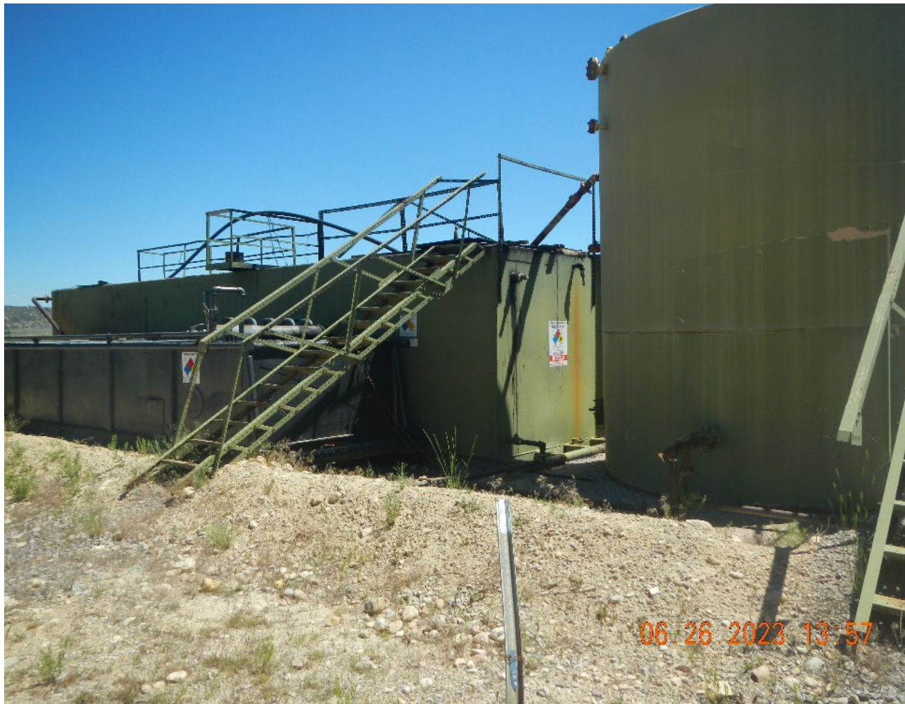
Photo #45 open top produced water treatment tanks.
