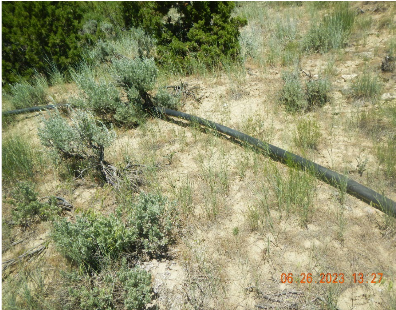
Photo #14 Flowline on surface, it appeared that no fluid was currently in this line.
