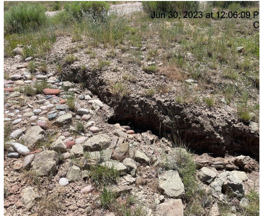
Photo # 2354 Rip Rap run needs maintenance (W/NW area of location)
