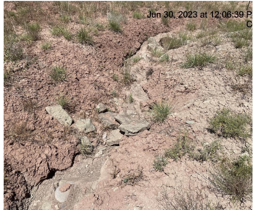
Photo # 2356 Check dams need maintenance (W/NW area of location)
