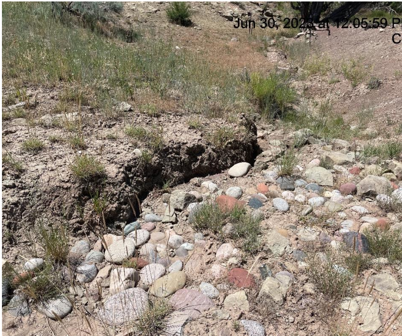
Photo # 2353 Rip Rap run needs maintenance (W/NW area of location)
