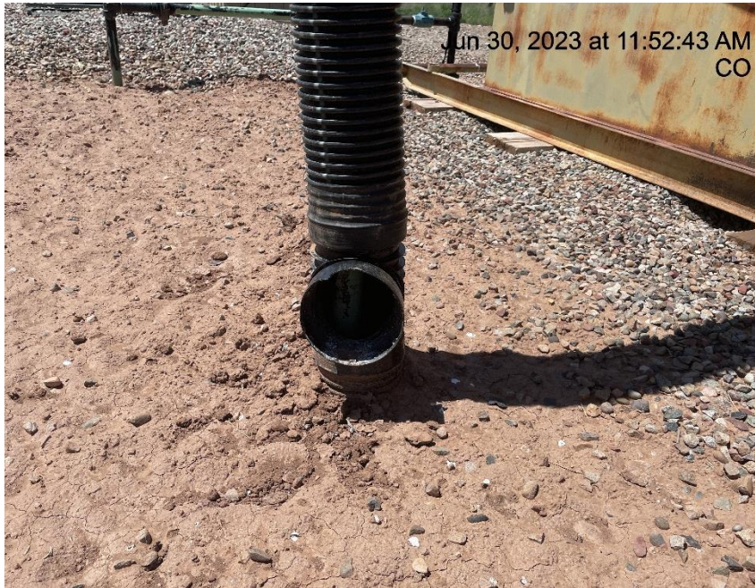
Photo # 2328 Flowline heating insulation open ended/wildlife hazard
