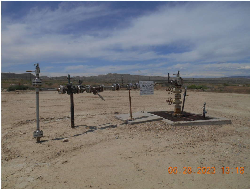
Injection wellhead
