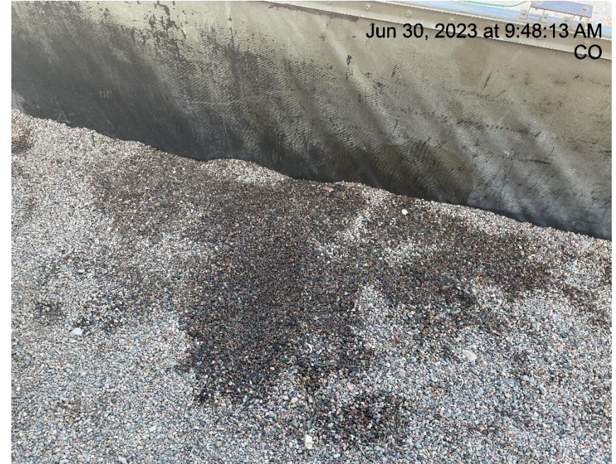
Photo # 2225 Stained gravel in secondary containment
