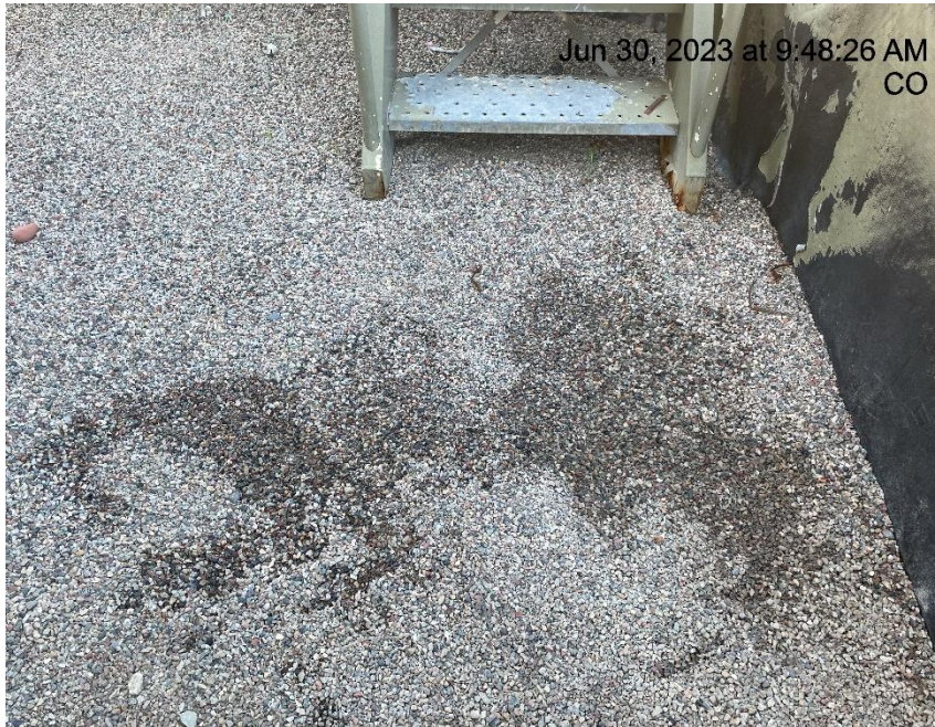
Photo # 2227 Stained gravel in secondary containment
