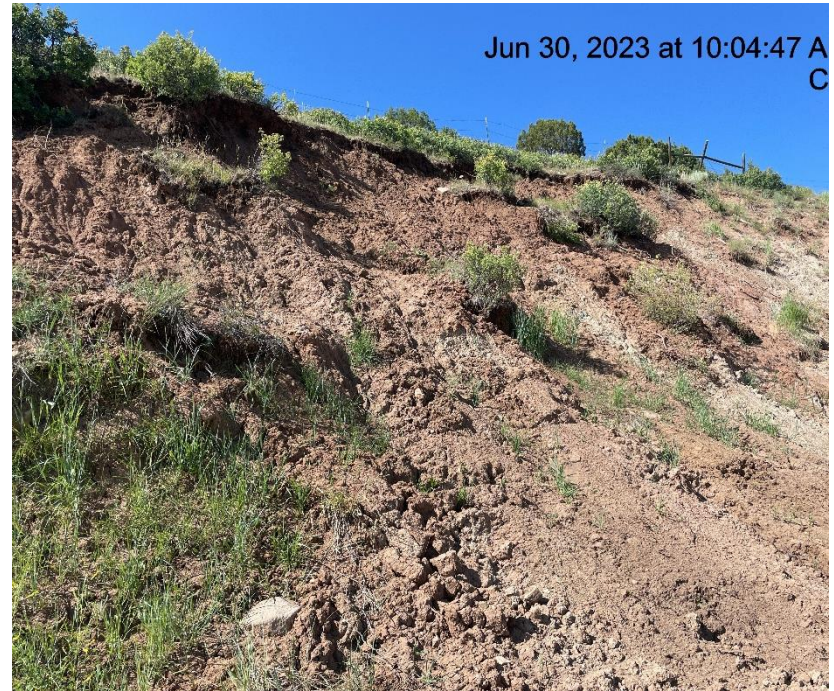
Photo # 2252 Lack of stabilization/erosion on cutslope along lease road
