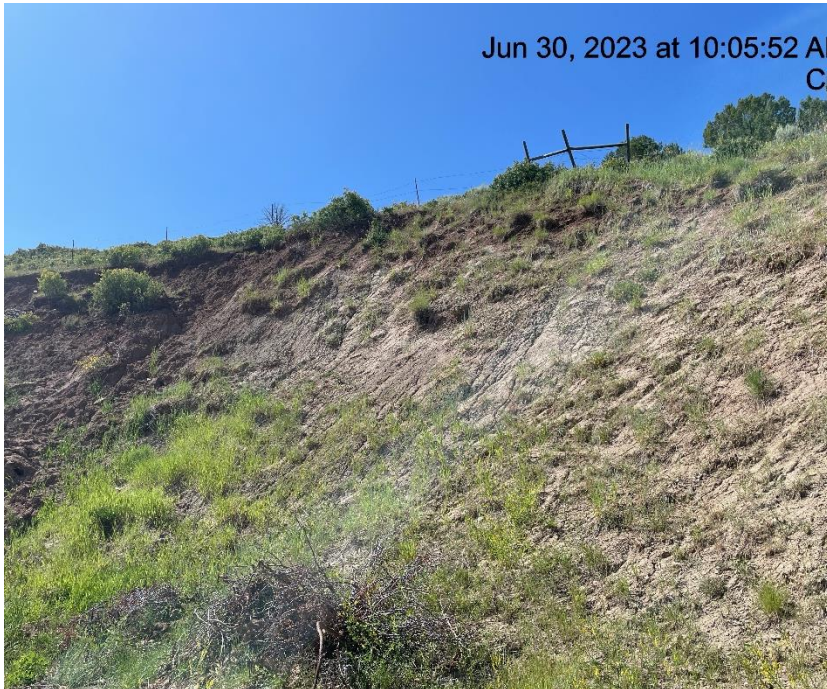
Photo # 2255 Lack of stabilization/erosion on cutslope along lease road
