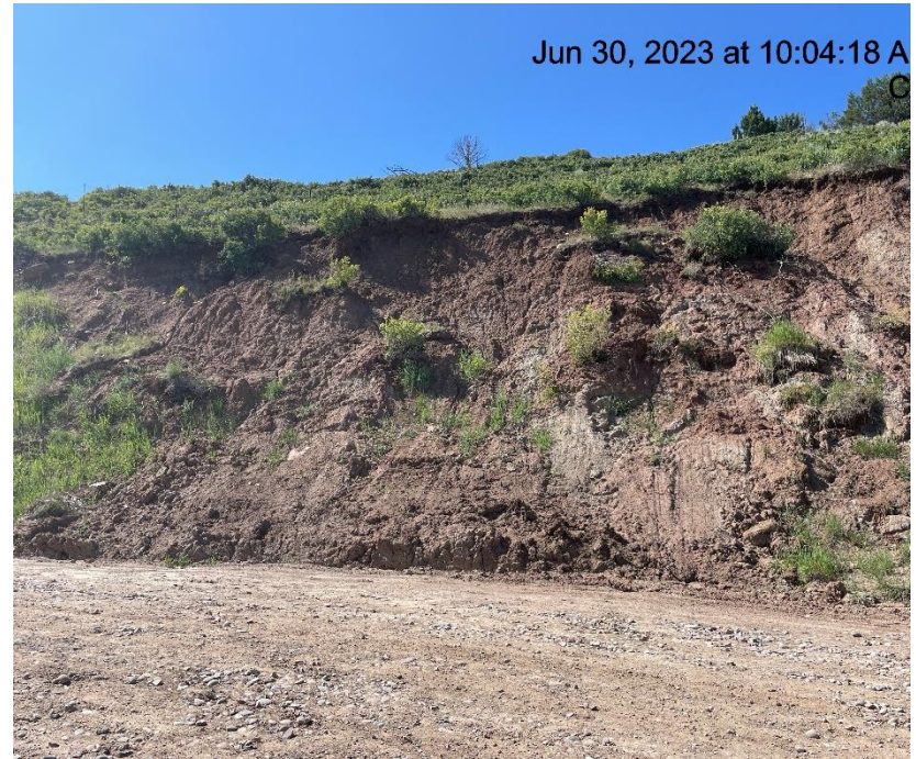
Photo # 2249 Lack of stabilization on cutslope along lease road
