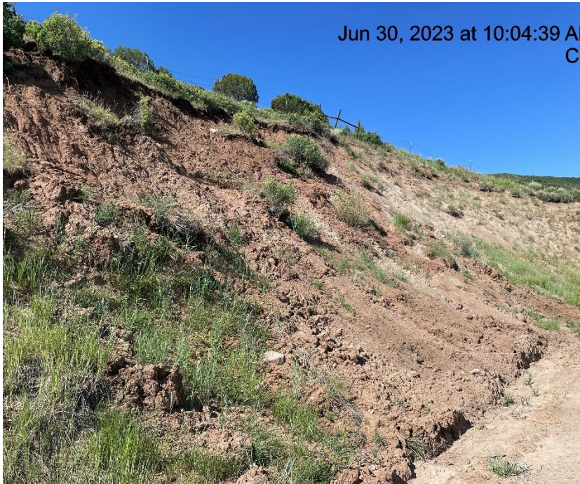
Photo # 2250 Lack of stabilization/erosion on cutslope along lease road
