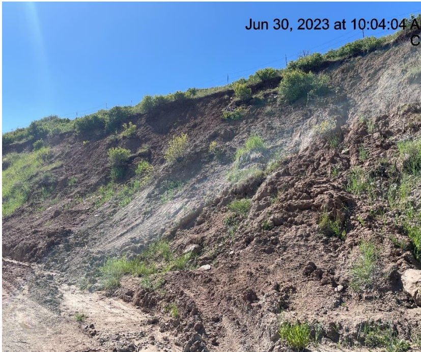
Photo # 2248 Lack of stabilization on cutslope along lease road
