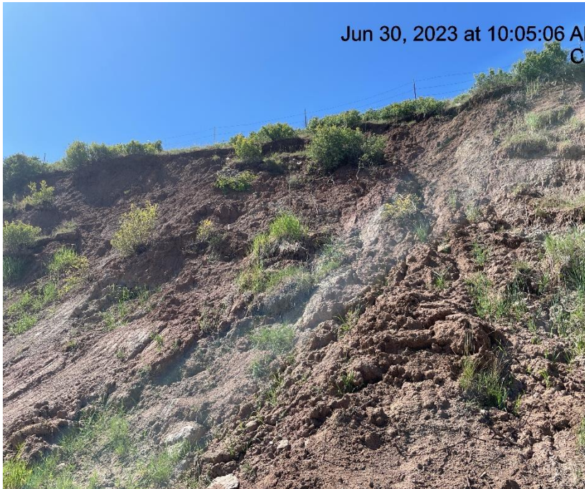
Photo # 2253 Lack of stabilization/erosion on cutslope along lease road
