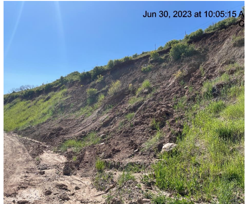
Photo # 2254 Lack of stabilization/erosion on cutslope along lease road
