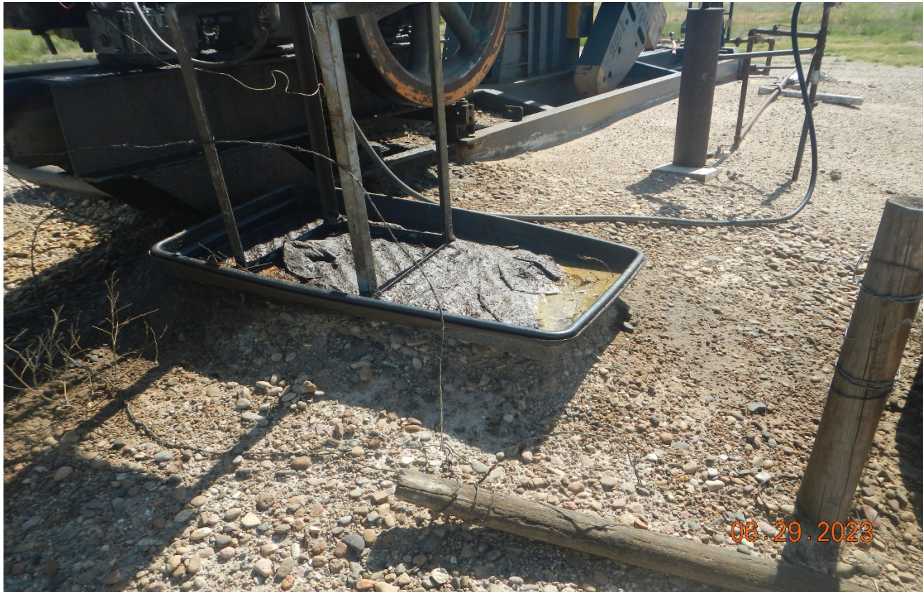
Photo 8. There is oily fluid in the containment next to the pump jack. Oily fluid has spilled onto the ground and needs to be cleaned up.
