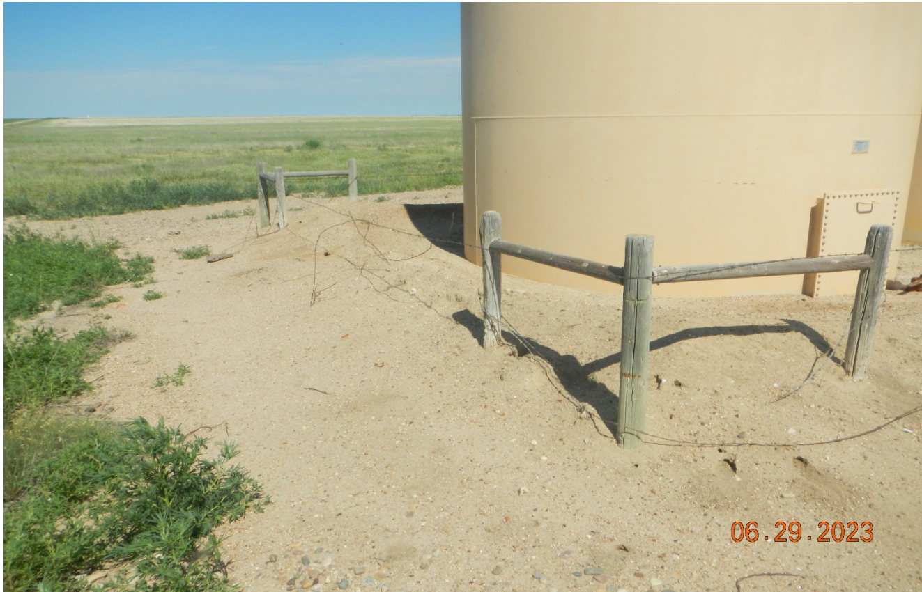
Photo 2. The fence around the tank is inadequate to prevent livestock entry and is not maintained. The berm around the tank is insufficient to contain a spill (150% of tank capacity) and has animal borrows the sides.
