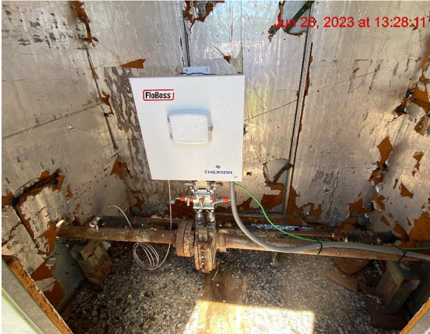
Gas Meter Calibration Record not Conspicuously Posted – Photo #04926
