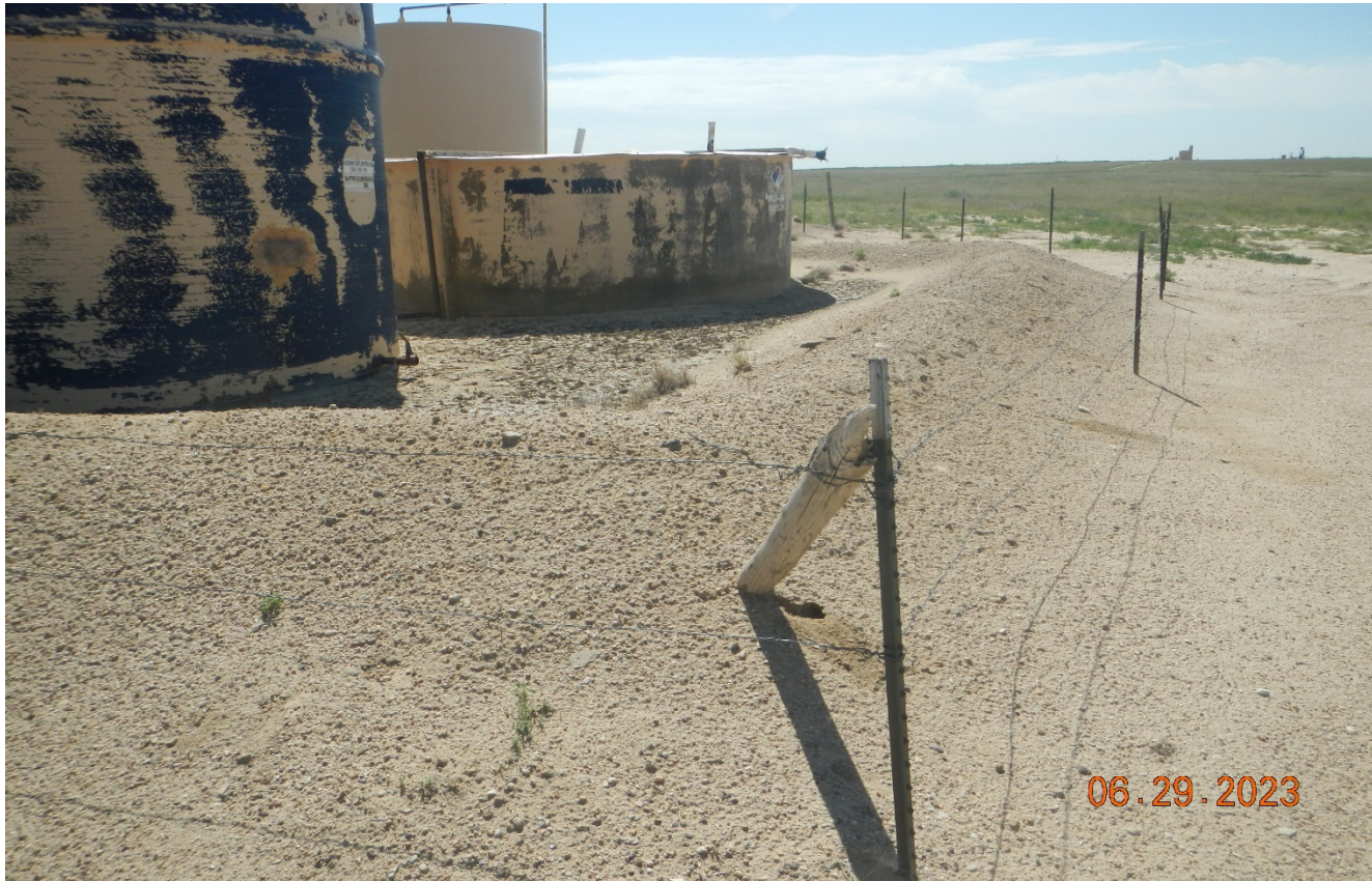
Photo 3. Facing at the backside of the open top tanks. The labeling on the tanks is missing and/or inadequate. The fence around the open top tank is inadequate to prevent livestock
