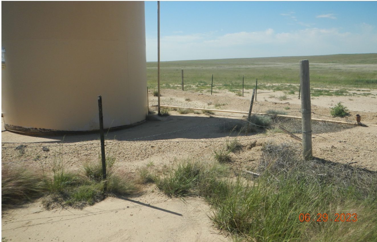
Photo 2. The fence around the tank is inadequate to prevent livestock entry and is not maintained. The berm around the tank is insufficient to contain a spill (150% of tank capacity).
