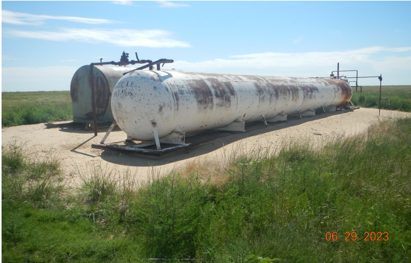
Photo 6. There is no labeling or secondary containment at these two large volume tanks.
