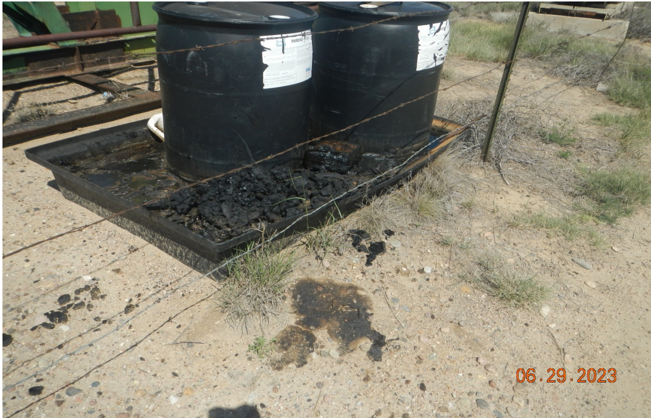
Photo 3. There is oily fluid and sludge that is overtopping the containment and needs immediate cleaned up and disposal.
