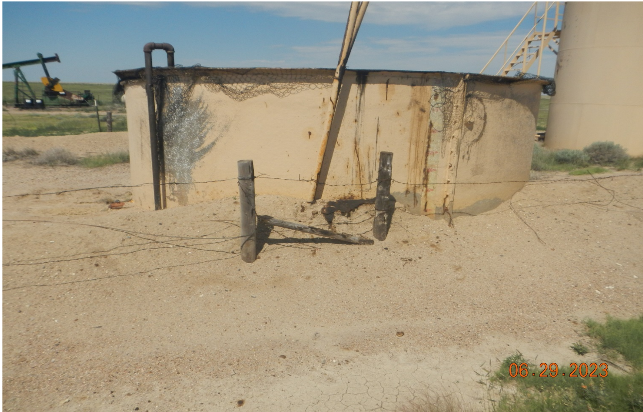
Photo 5. There is oily sludge that has overtopped the tank and berm. The berm is inadequate to contain a spill.
