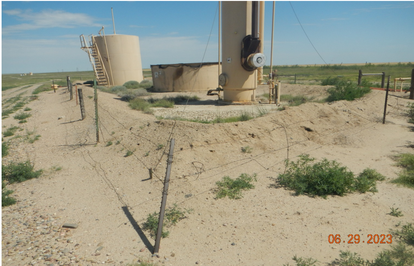
Photo 4. The fence around the tank battery is inadequate to prevent livestock entry and is not maintained. The berm around the tank has animal borrows and is compromised.
