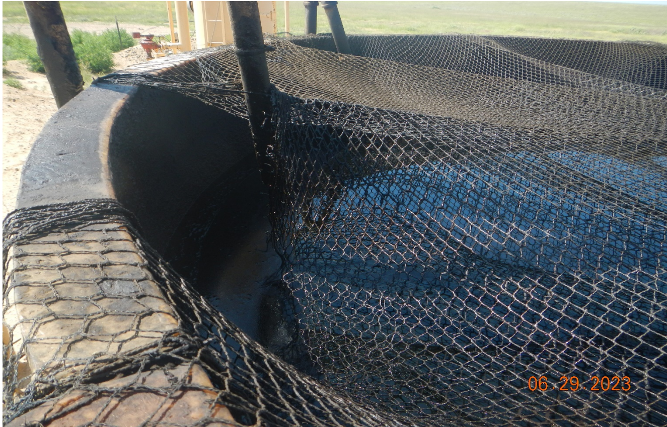
Photo 6. The netting on the open top tank is in disrepair.
