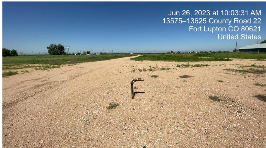
**Photo 4. Photo taken of pipe riser unmarked, unlabeled and unprotected from traffic.**
