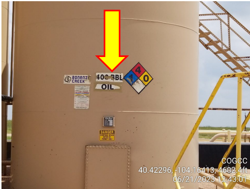
Photo 9 – South Tank – Capacity and Content Labels
