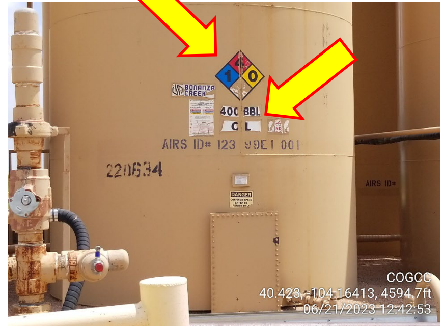
Photo 8 – Middle Tank – NFPA, Content, and Capacity Labels
