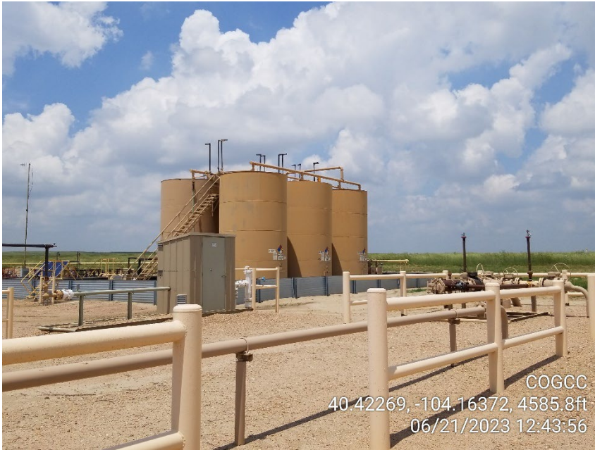
Photo 13 – Gas Meter and Tank Battery
