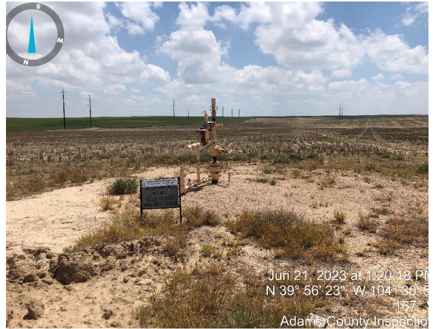
Photo# 4 Well head.
