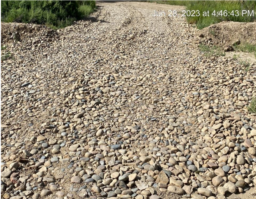
Tracking pads installed at entrance to location.
