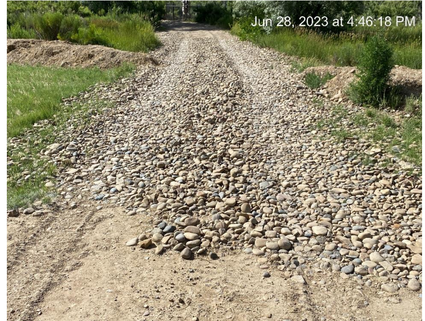
Tracking pads installed at entrance to location.
