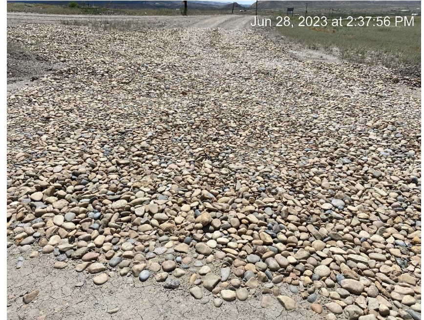
Tracking pad installed at Southwest location entrance since last inspection.
