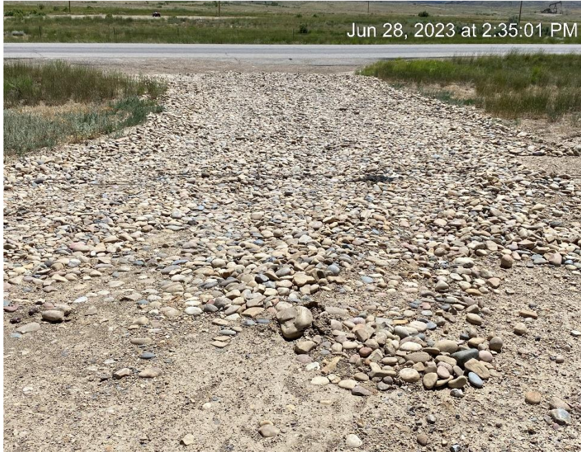
Tracking pad installed since last inspection off Hwy 64.
