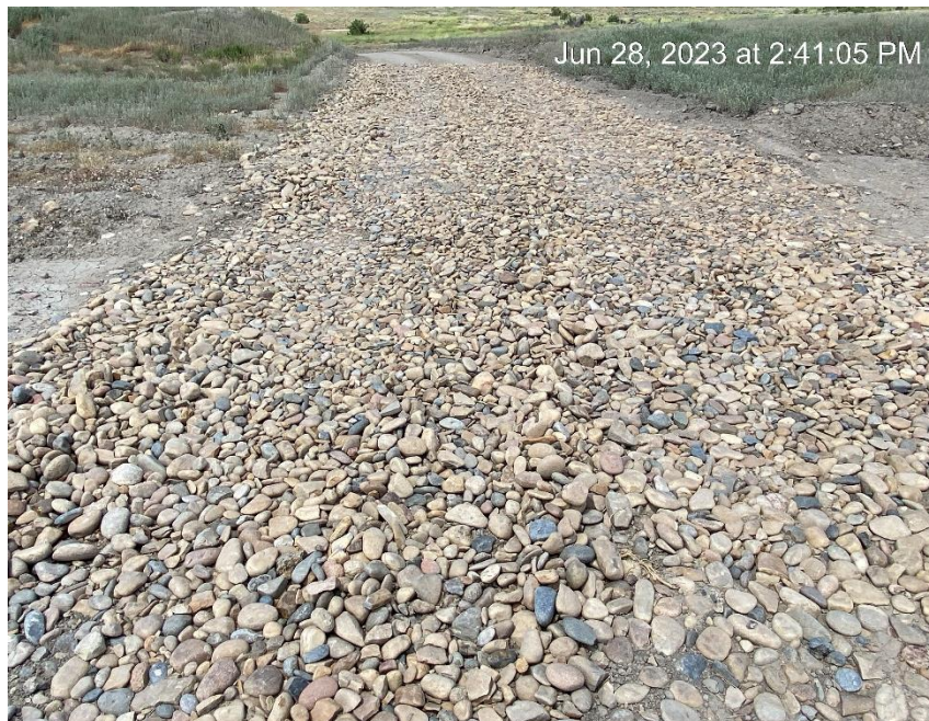
Tracking pad installed at Northwest location entrance since last inspection.
