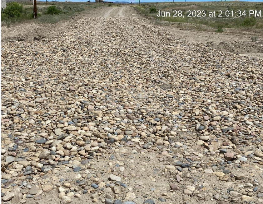
Tracking pad installed since last inspection.
