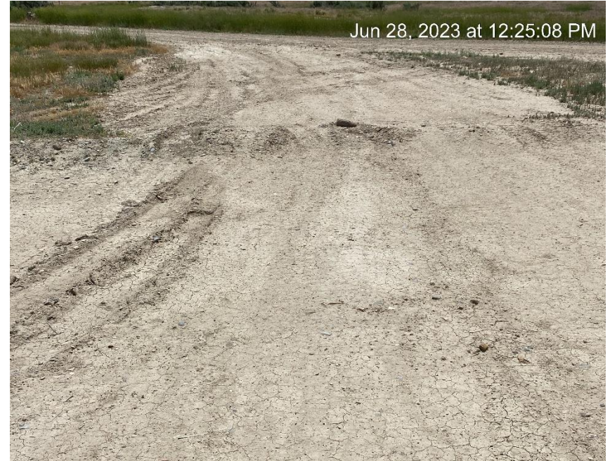
No BMPs to control vehicle tracking at Southeast location entrance
