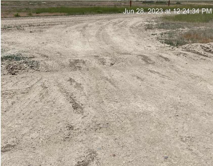
No BMPs to control vehicle tracking at Northeast location entrance
